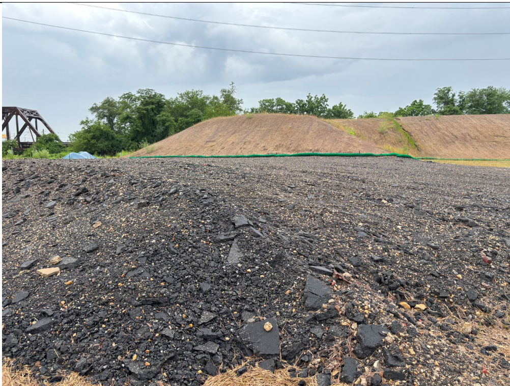
Asphalt millings in downslope portion of site.
