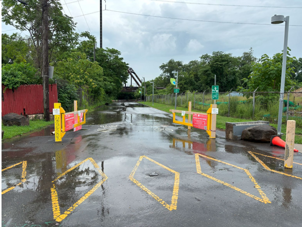
Open gates at corner of 51 st and Botanic Sts., with warning signage still present, adjacent to downslope boundary of site.
