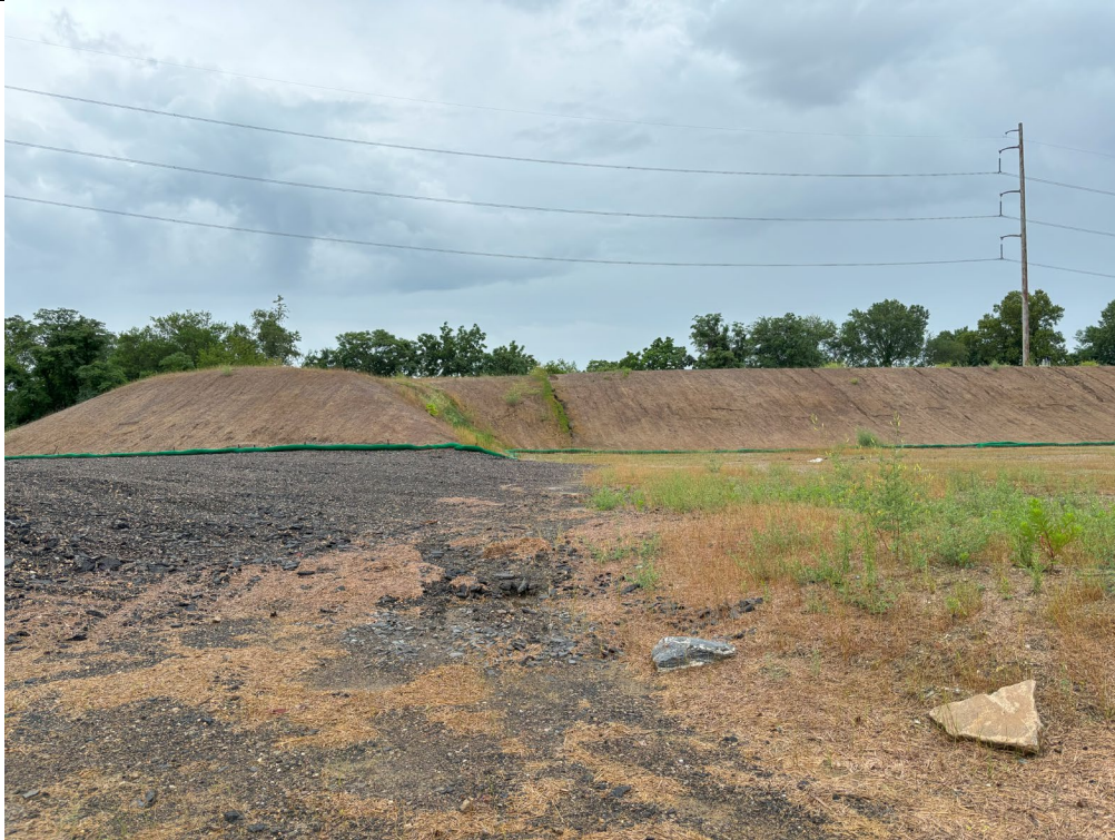
Large fill dirt stockpile in distance, with some partially stabilized earth at right.
