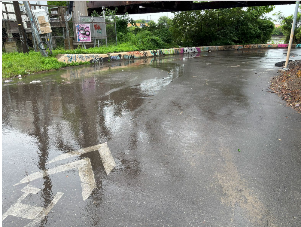
Bartram's Garden trail with stormwater, and previous sediment staining at bottom right.
