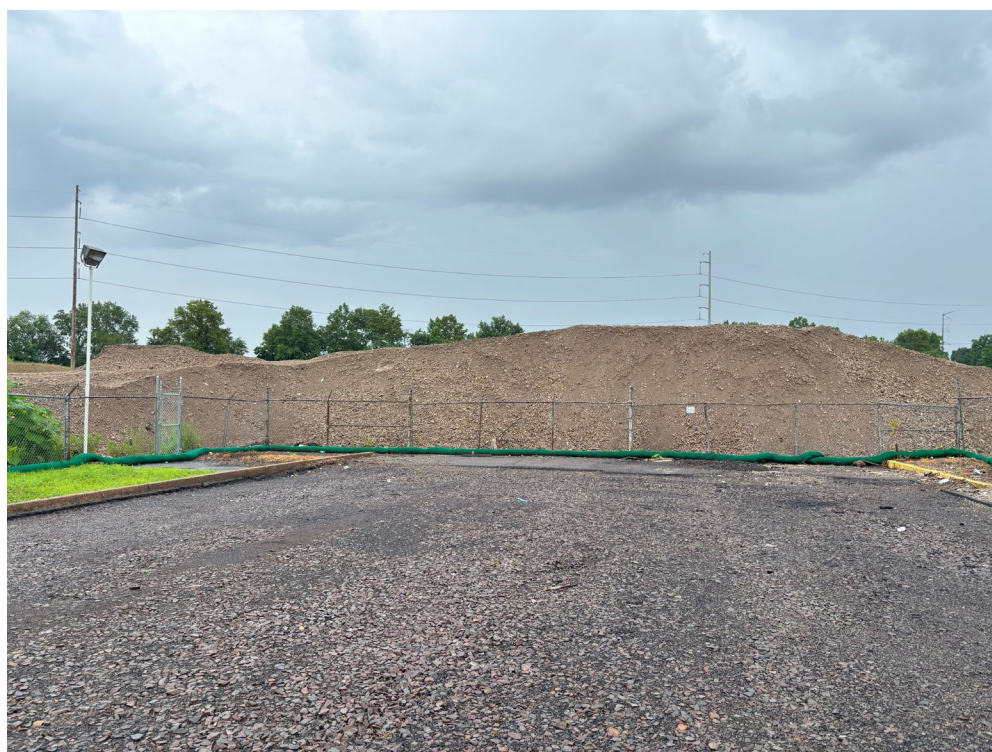
Stone stockpile and midslope filter sock.
