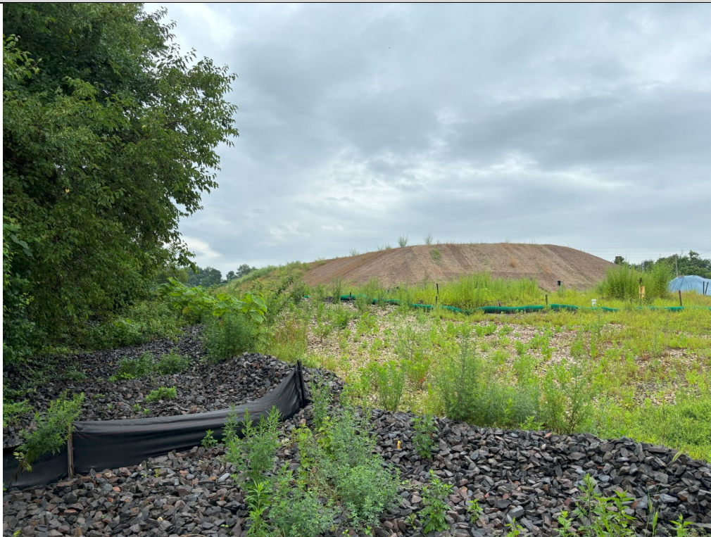
Downslope and back side of large fill dirt stockpile (adjacent to train tracks); rock-covered swale and silt sock at left.
