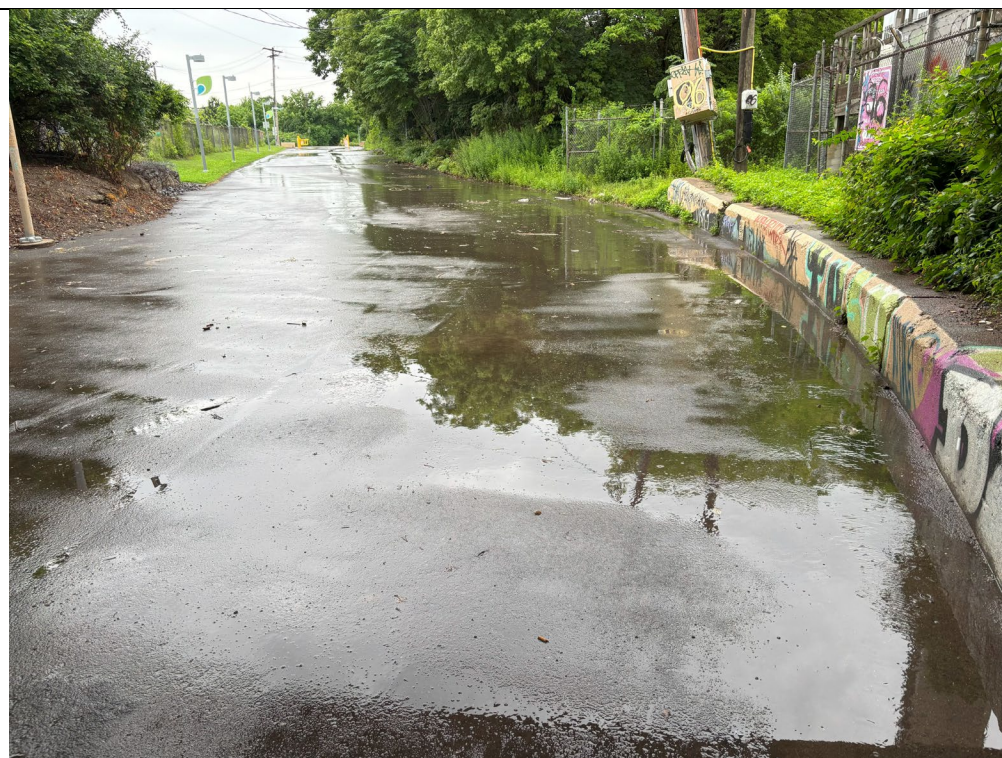
Bartram's Garden trail with stormwater, looking upslope from under railroad bridge towards Site.
