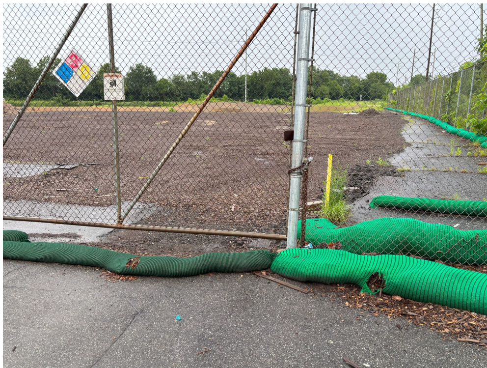
Upslope gate filter sock and upslope section of site.
