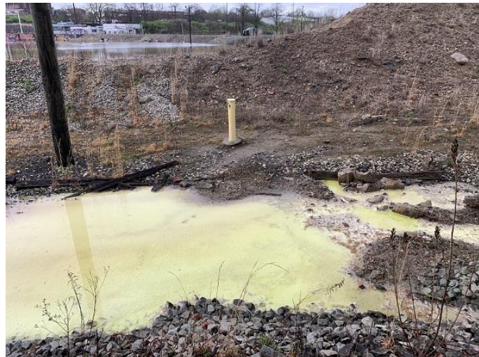
Pooled material in the ditch near MW-3
