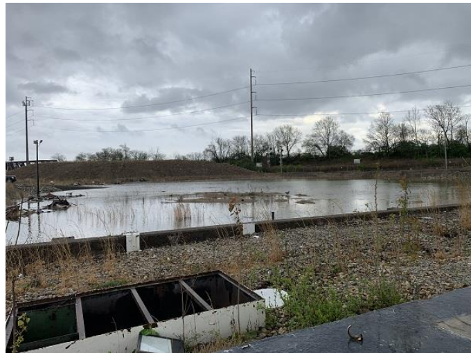
Empty tank containment looking east
