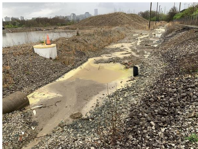
Discoloration at the concrete pipe discharge point
