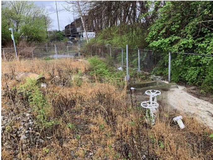
Eastern corner separator and ditch
