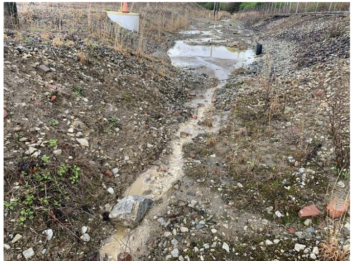
Ditch, concrete pipe discharge and valve box
