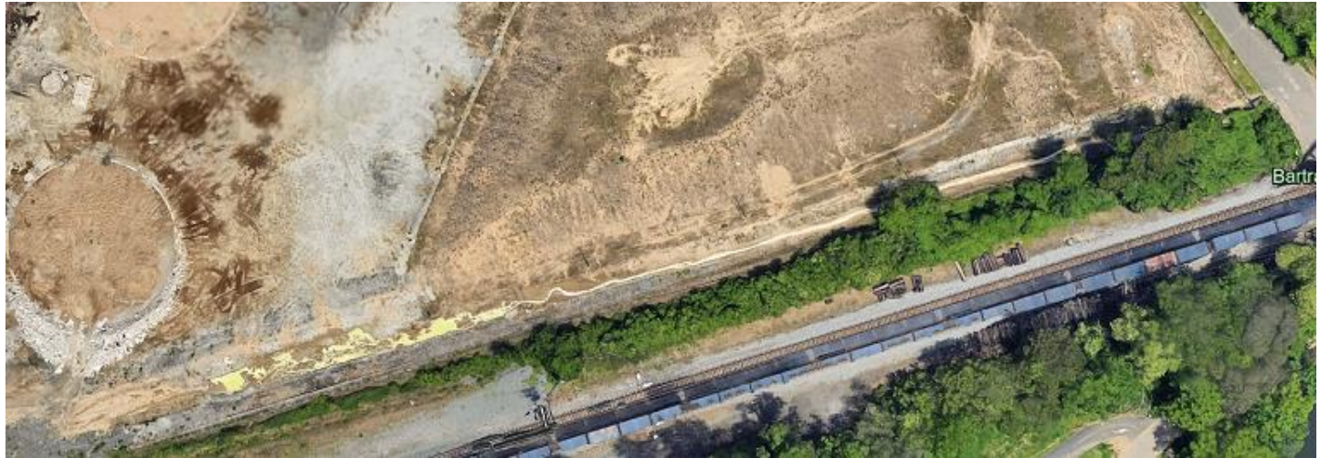
5/10/23 Google Earth view of the ditch showing discoloration
