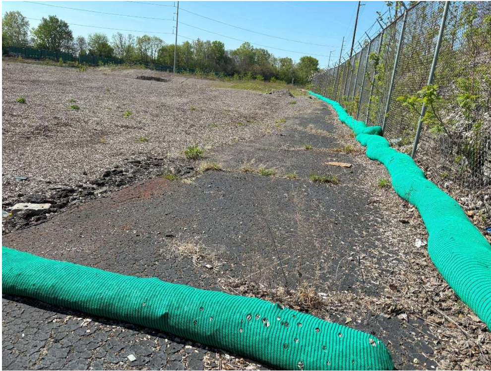
Filtersock and upslope mulching of site.
