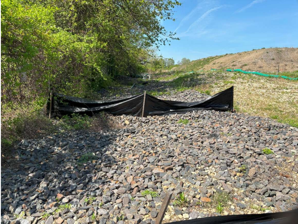
Rock-covered swale and silt fence.
