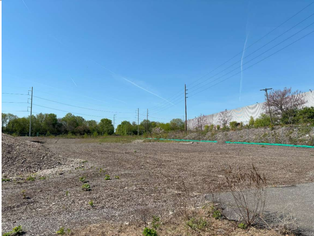
Mulching of upslope portion of site.
