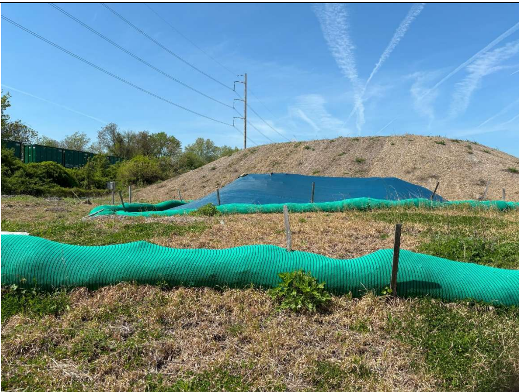
Downslope filter sock and covered contaminated fill dirt stockpile.
