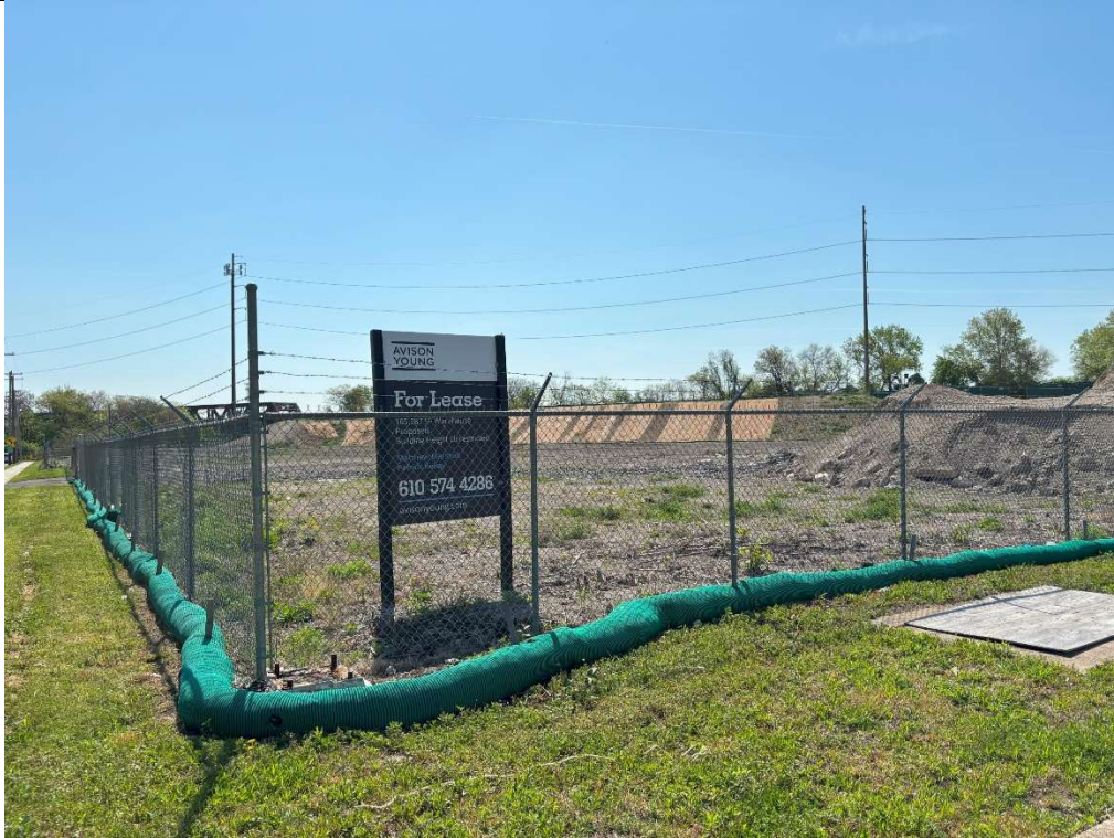
"For Lease" signage and midslope filter sock facing 51 st St.
