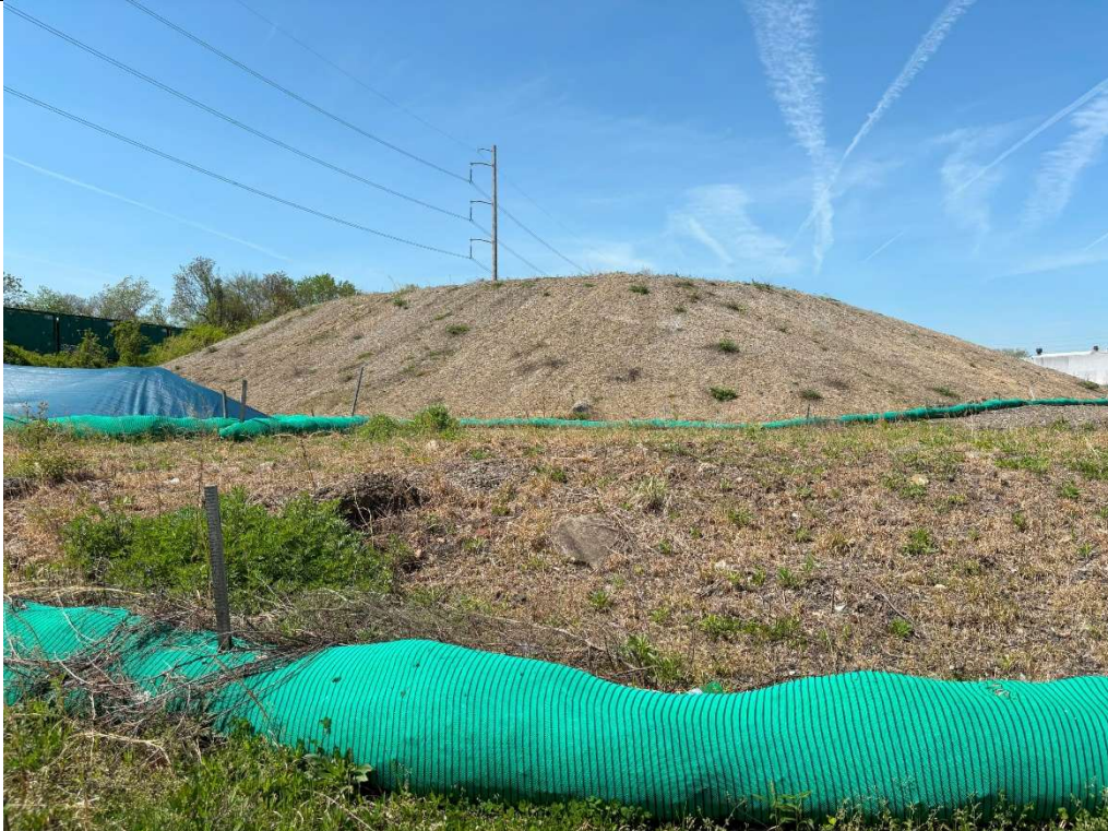
Downslope filter sock and downslope end of large fill dirt stockpile.
