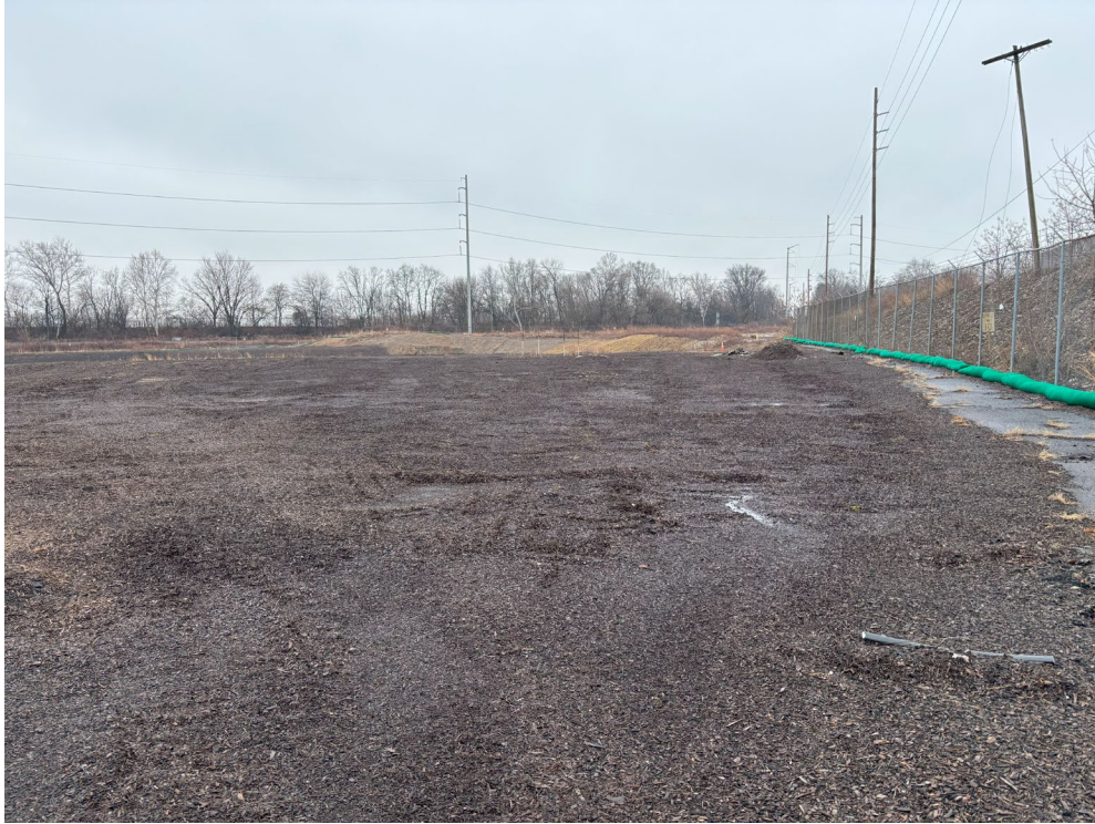
Mulched upslope portion of site.
