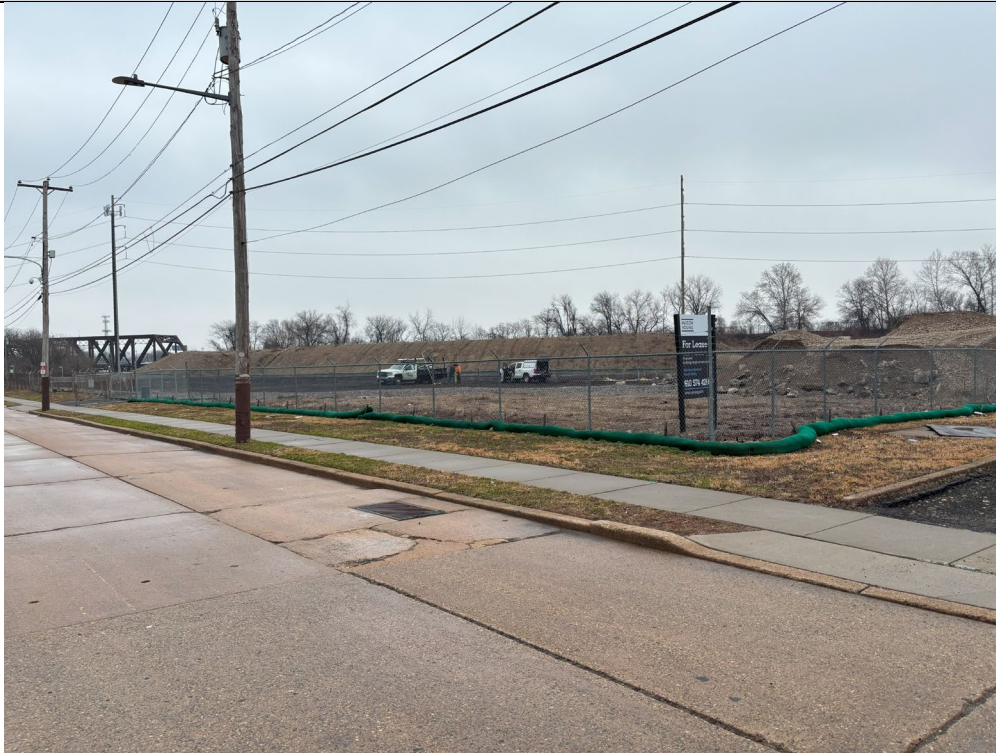
Filter sock, mulch, and "For Lease" signage with large fill dirt stockpile and well drilling persons and equipment in distance.
