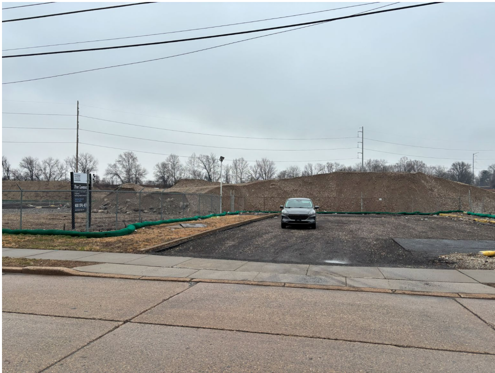
Stone stockpile and filter sock in middle portion of site along 51 st St.
