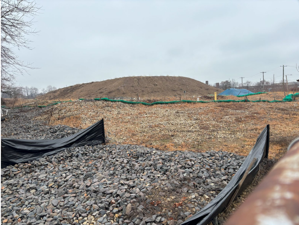
Downslope and rear portion of large fill dirt stockpile with rock-lined swale and silt fence in foreground.
