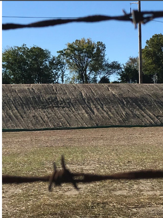
Erosion gullies visible on the large fill dirt stockpile.
