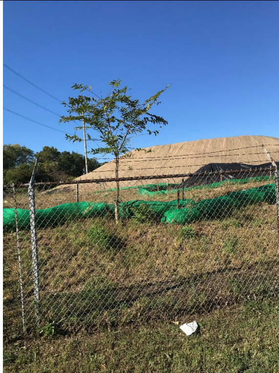
Most downslope portion of large fill dirt stockpile, with smaller tarped pile of contaminated dirt in front.
