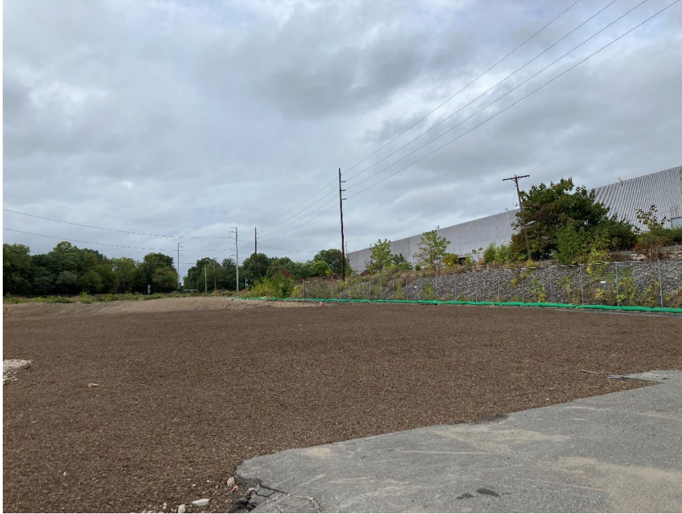
Completed mulching of upslope portion of site.
