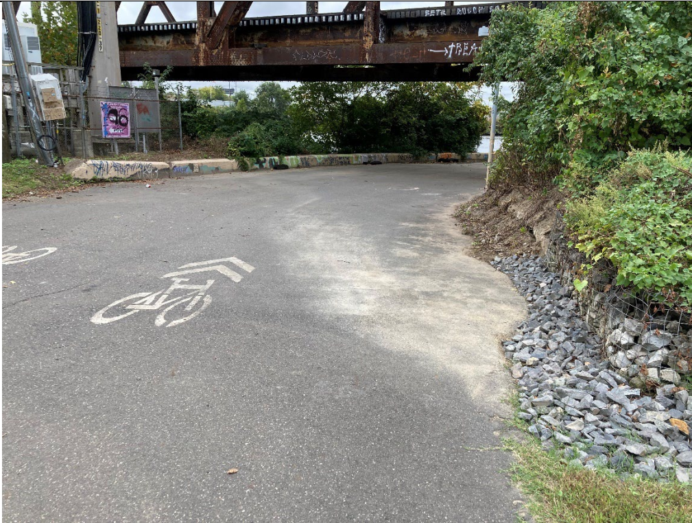
Sediment staining on Bartram's Garden trail, looking downslope towards railroad bridge.
