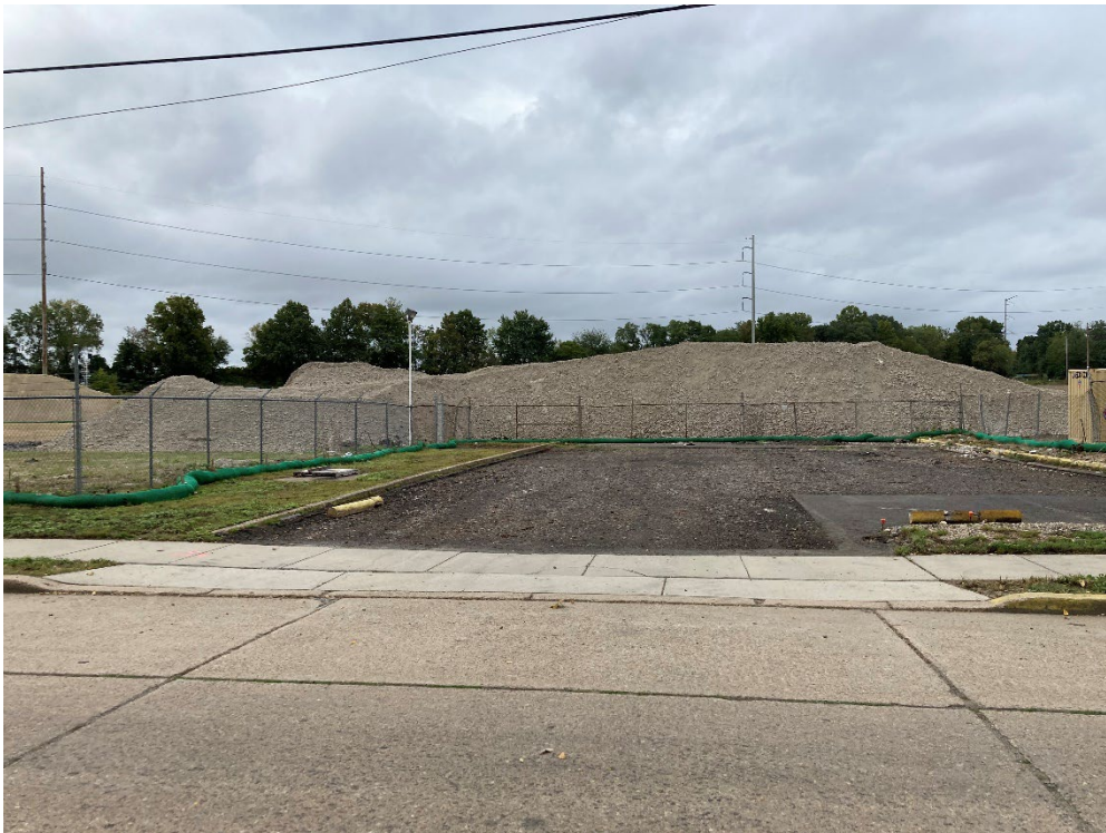
Large rock and gravel stockpile in middle section of site along 51 st St.
