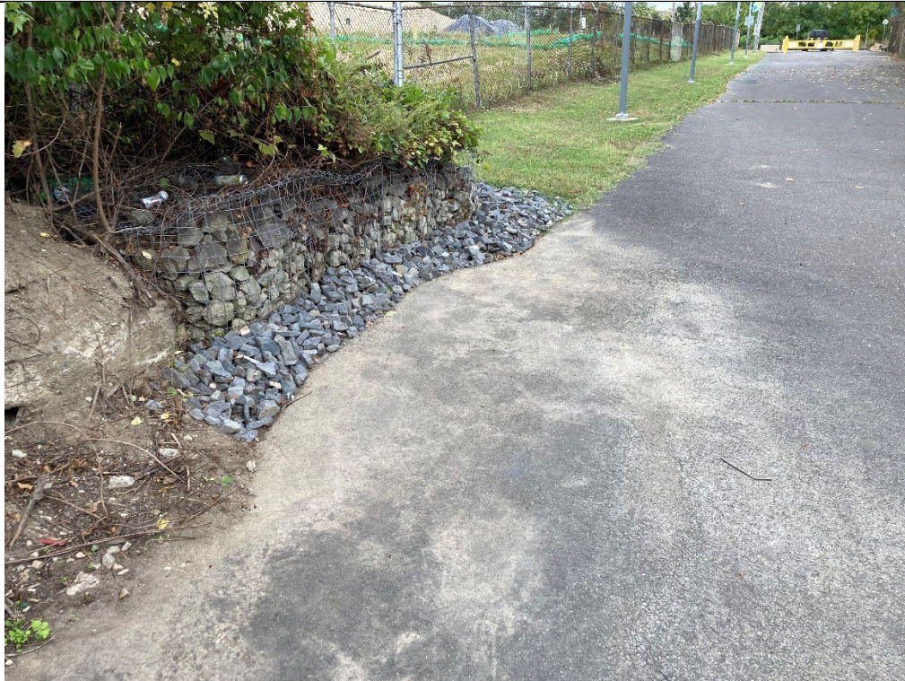
Sediment staining on Bartram's Garden trail.
