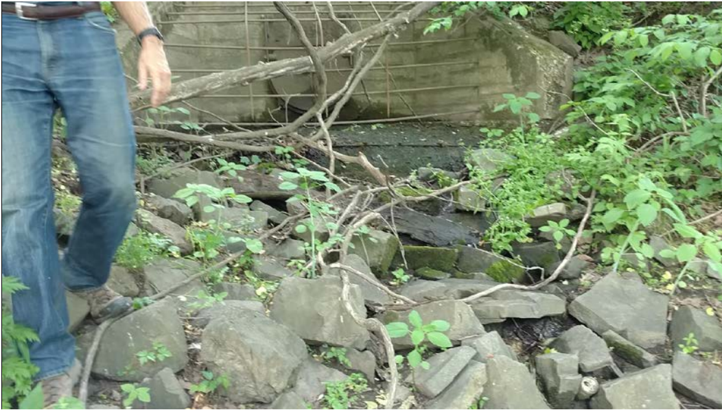
Photograph No. 4 Facing south/southwest at Outfall #3
