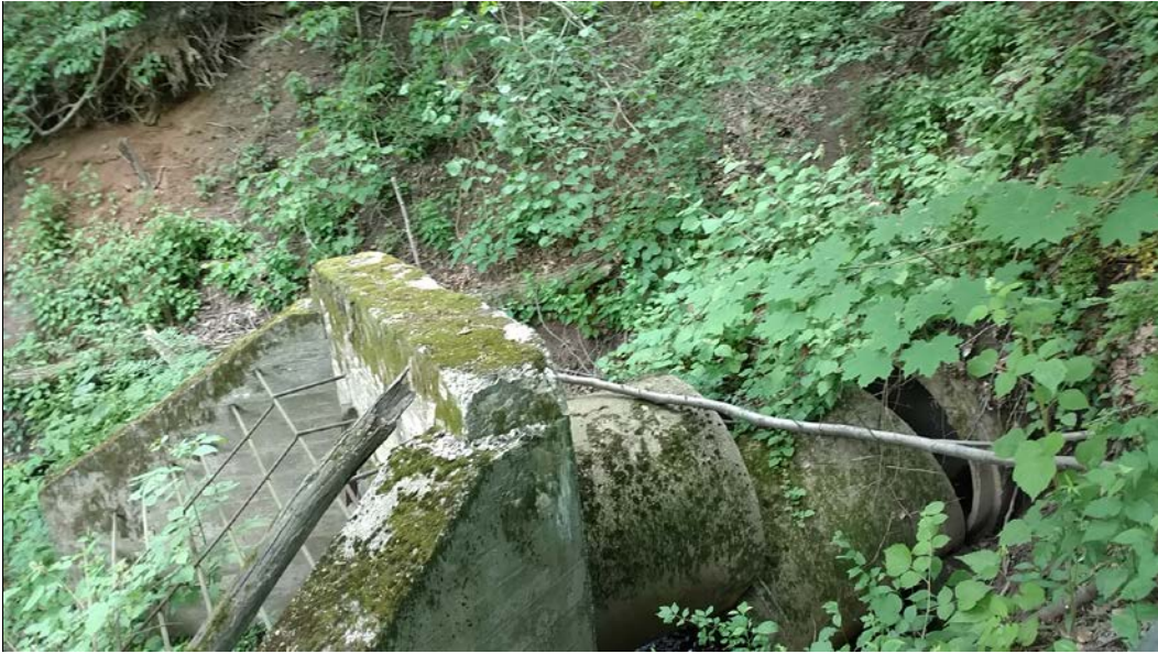
Photograph No. 5 Facing south/southeast at Outfall #4
