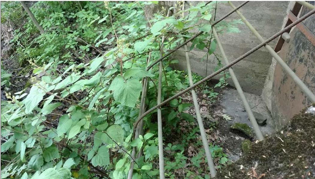
Photograph No. 6 Facing south at Outfall #4
