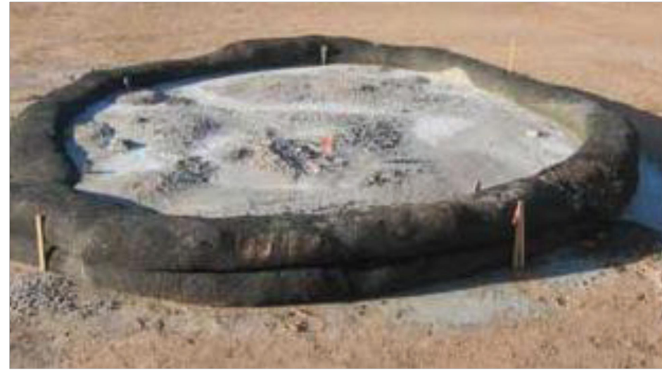
FIGURE 3.18 Typical Compost Sock Washout Installation
