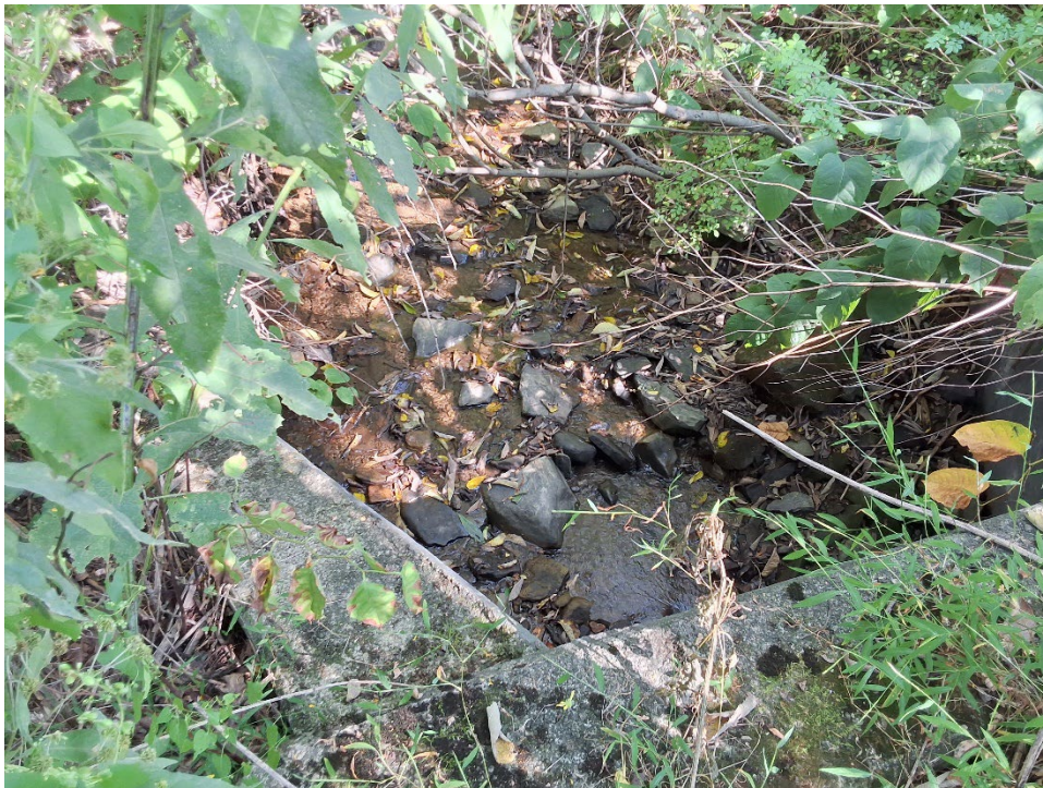
Photograph 10 –View of stream S-01 (Trib 44075 to Two Lick Creek) from an existing bridge in western portion of the study area (facing upstream).
