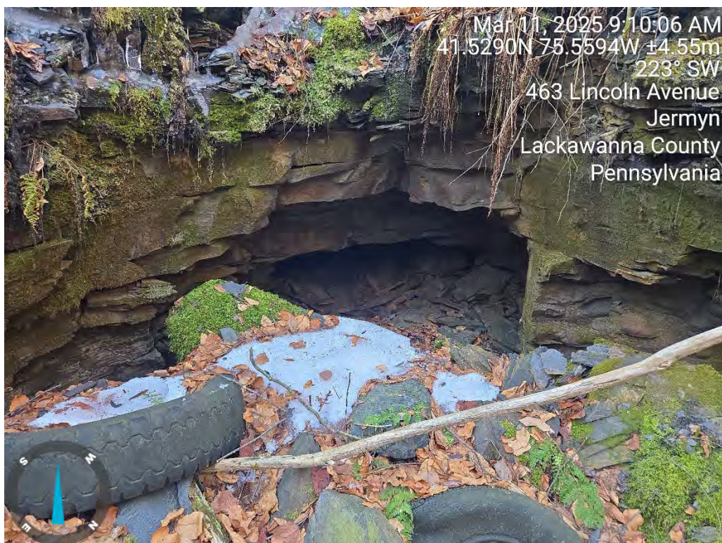
Photograph 14 illustrates a collapsed deep mine entrance. The view is facing southeast.
