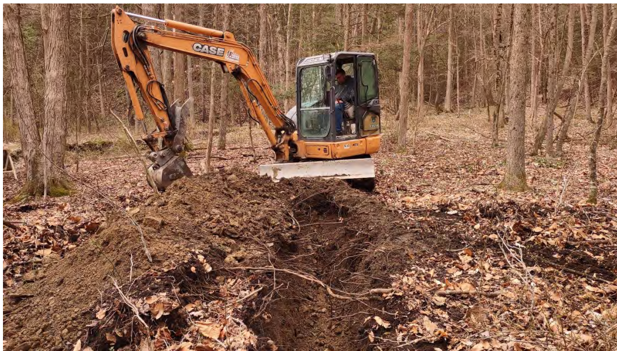
Figure 16. The hydraulic excavator at Trench 1.
