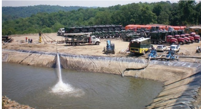
Above: Flowback pit. (Source: U.S. DOE/NETL) Right: Flowback tanks. (Source: U.S. EPA)
