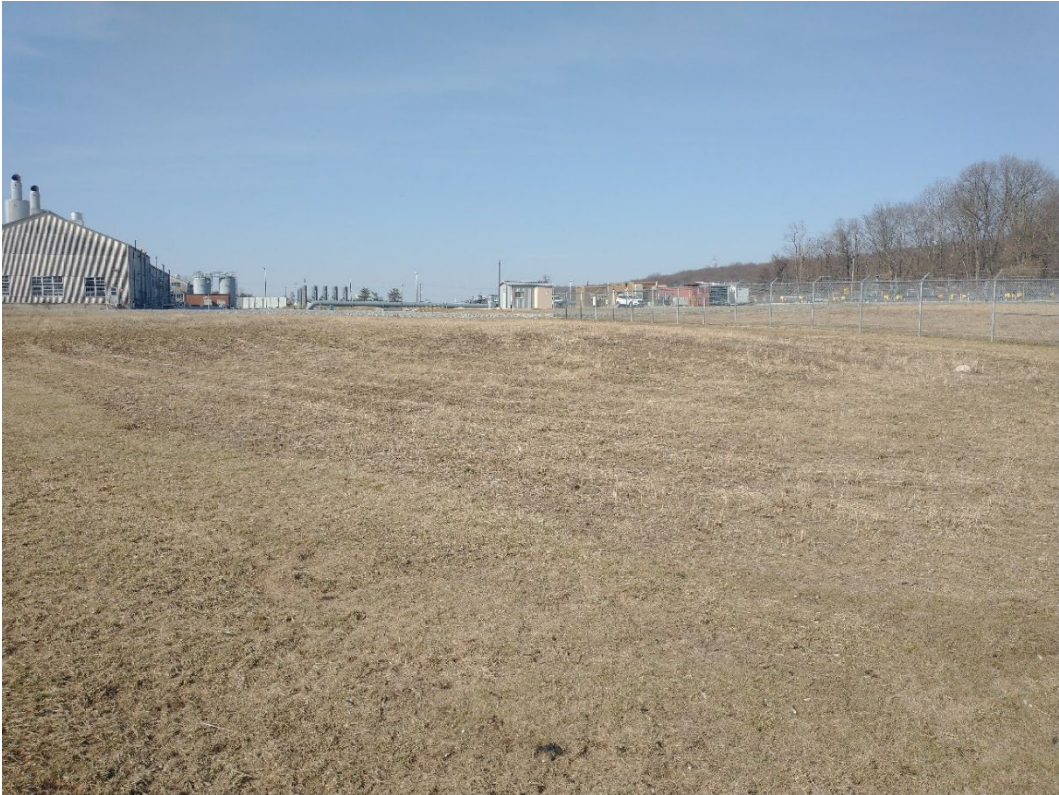
Photo 1: Existing Area at Proposed Level Spreader and Riprap Apron
