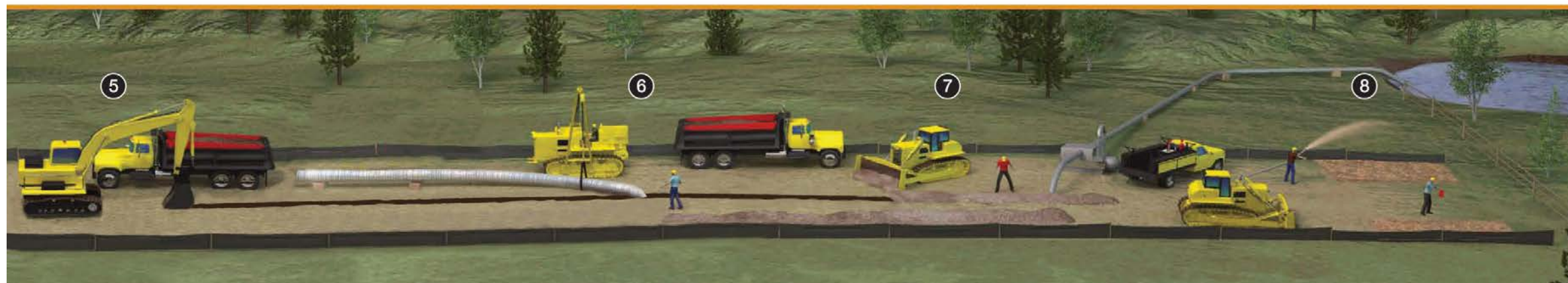
Figure 1.3-1 Typical Pipeline Construction Sequence
