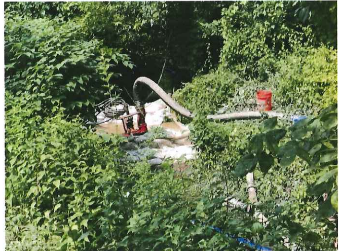
IR Location in UNT to Chester Creek – Sandbag Containment & Pump
