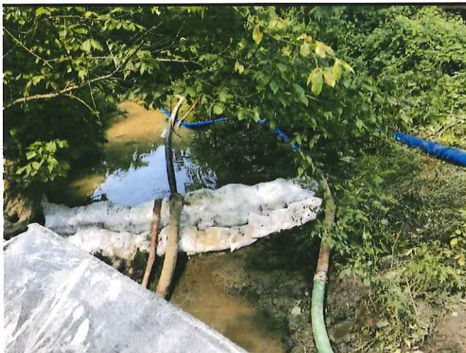
Coffer Dam and pump around in UNT to Chester Creek
