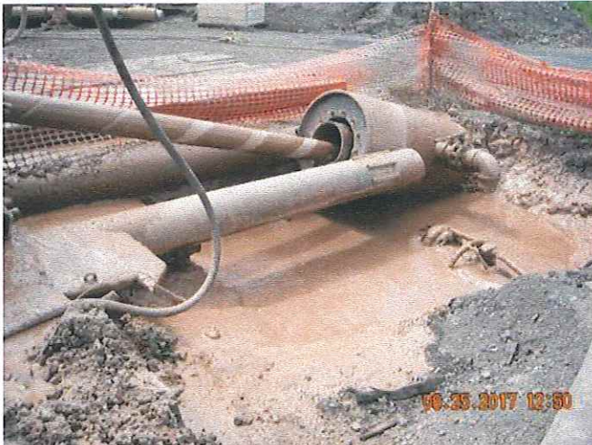
East Shore HDD Mud Pit (Highspire Borough, Dauphin County)
