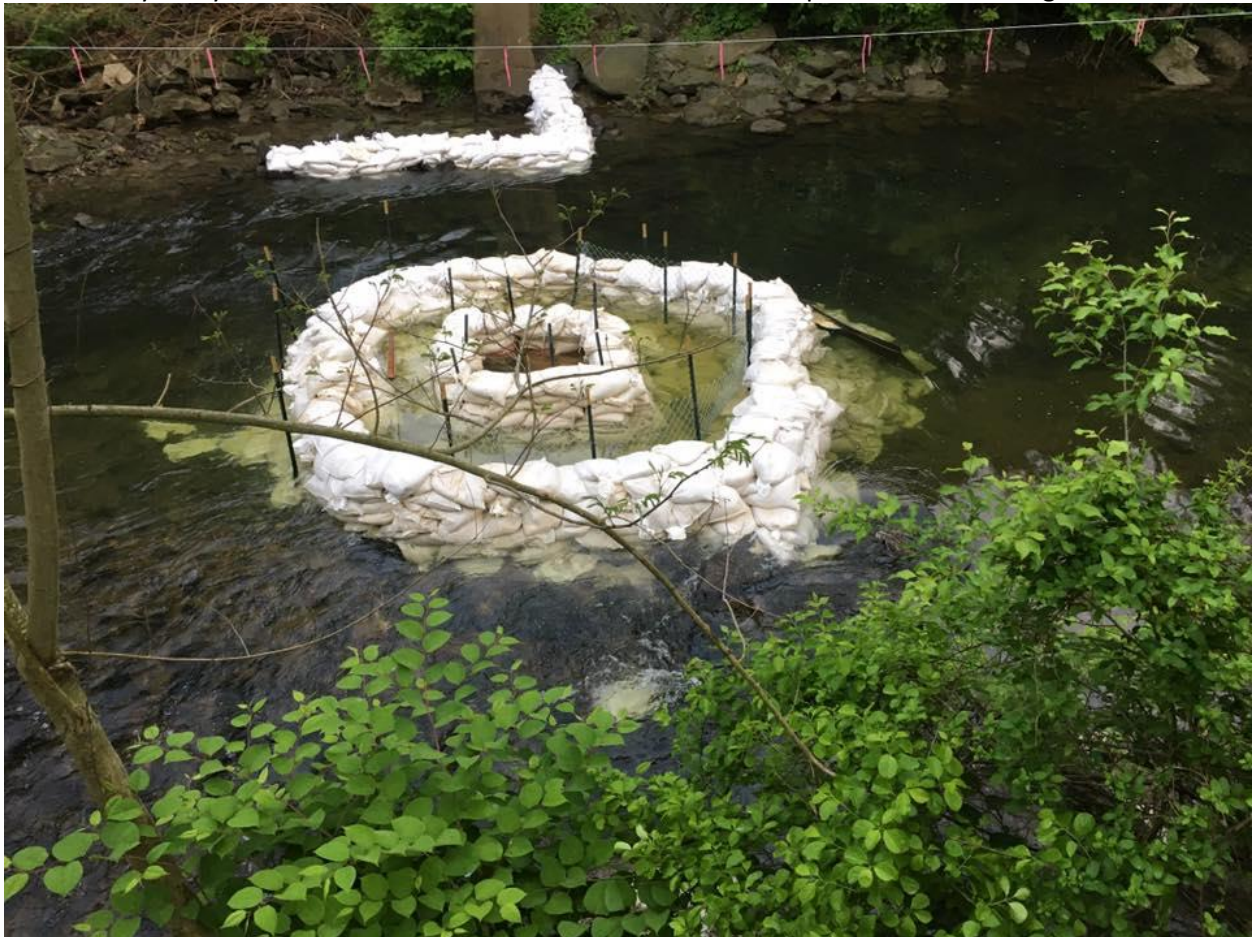
Large walls of sandbags placed in center of Chester Creek. Image by area resident.
