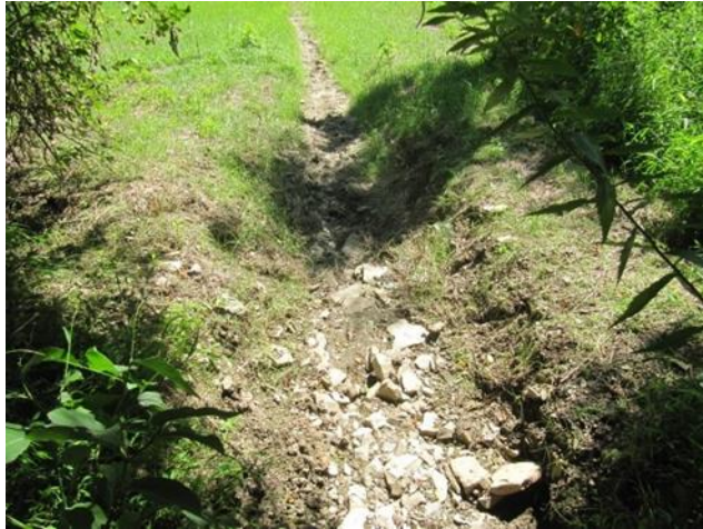
Photo No.: 13 Direction: Upstream Comments: S-096
