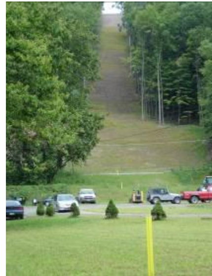
Completed Gathering Line & Right-of-Way – Eaton Twp., Wyoming County
