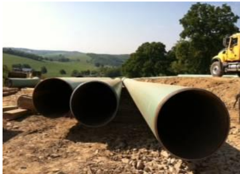
20" Pipelines Awaiting Installation – Smith Township, Washington County
