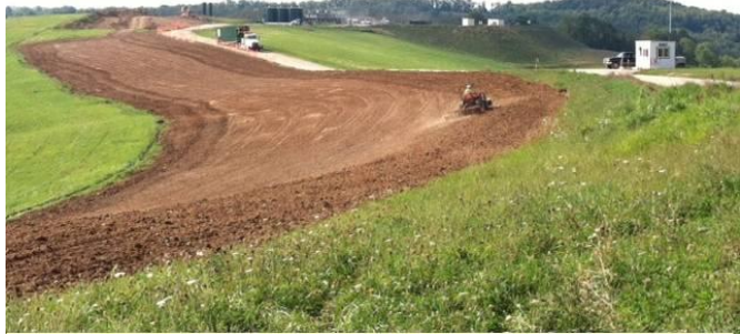
Right-of-Way Reclamation Smith Township, Washington County
