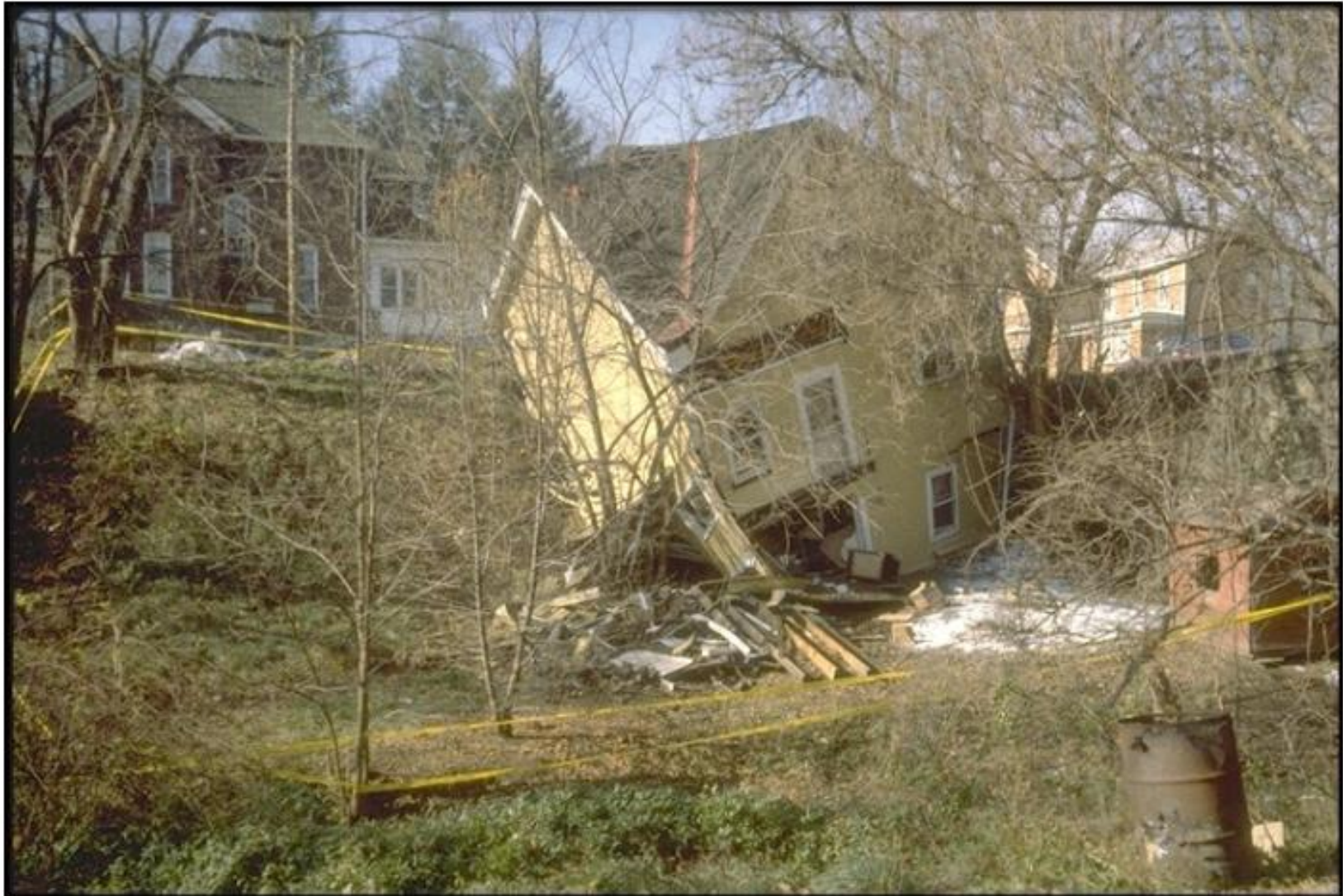
FOUNDATION FAILURE
