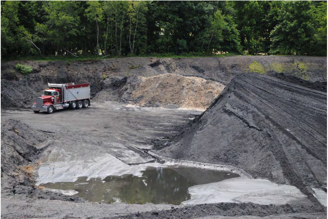
Removing material from the lower level basin AMLF-05 looking Southwest. Date: 7/15/19
