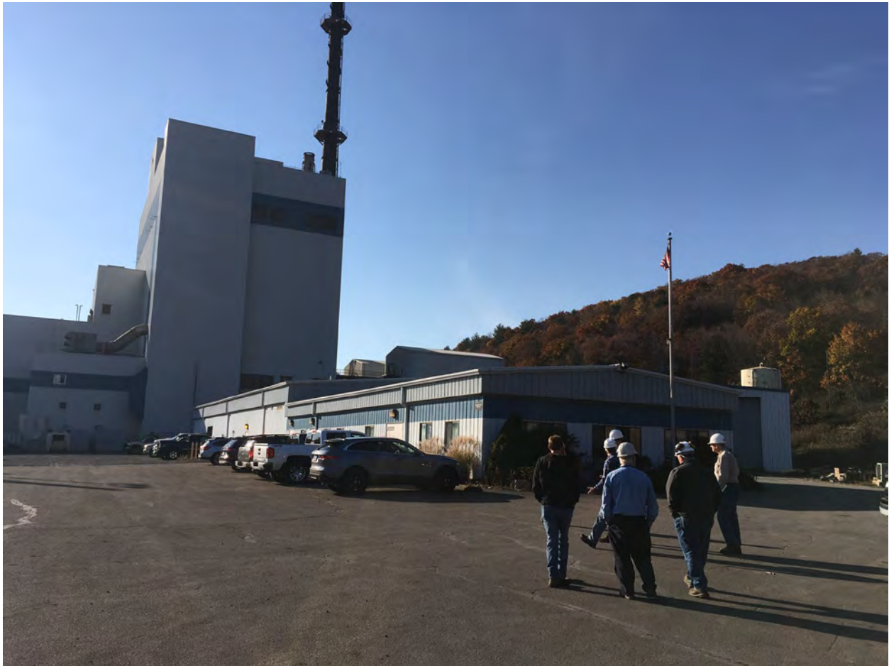
Visit to Panther Creek CoGen Plant on 11/9/2021
