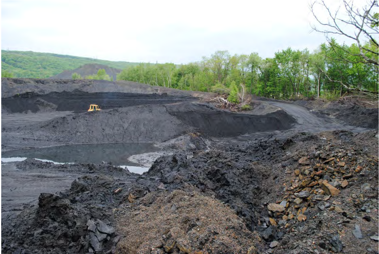
Bulldozer mounding material for onsite transport in AMLF-05 looking north, Date: 05-17-19
