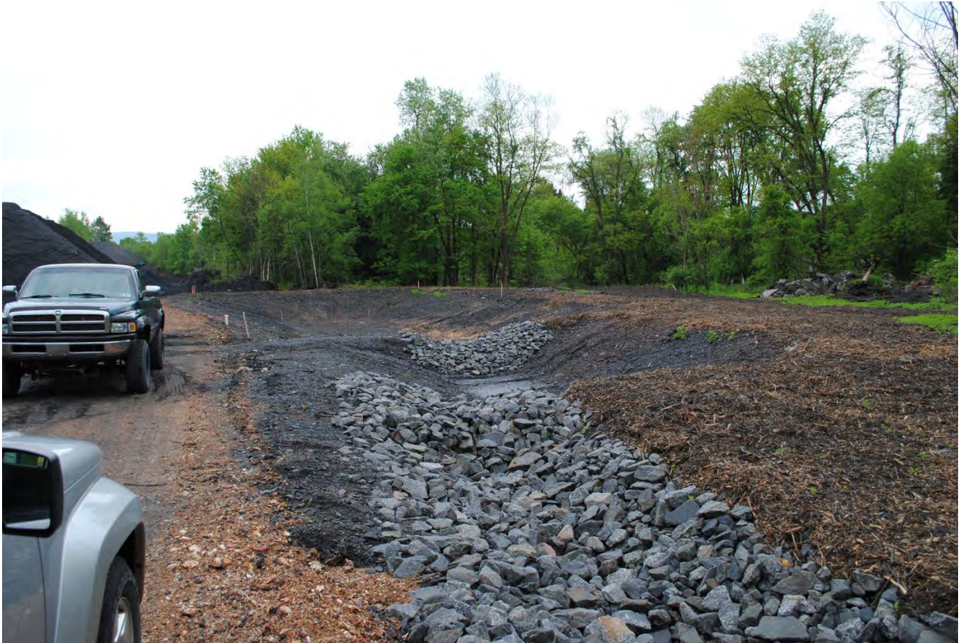
E&S drainage channel and basins looking south, Date: 05-17-19
