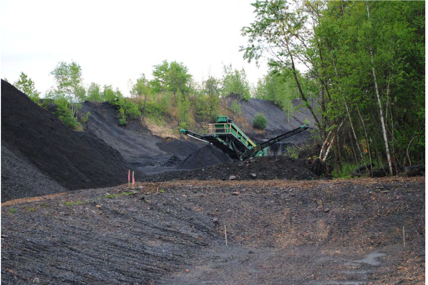
Material Processor near loading area, Date: 05-17-19
