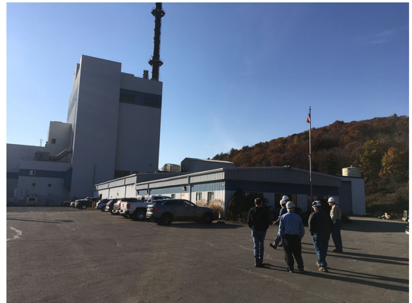
Panther Creek CoGen Plant Nesquehoning, PA Carbon County
