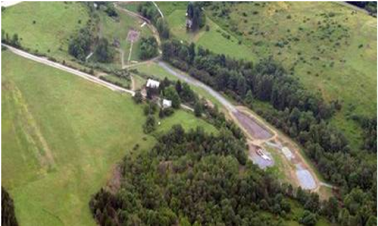
Figure 19. Completed passive mine drainage treatment system in the Porcupine Hollow Tributary of Dents Run.
