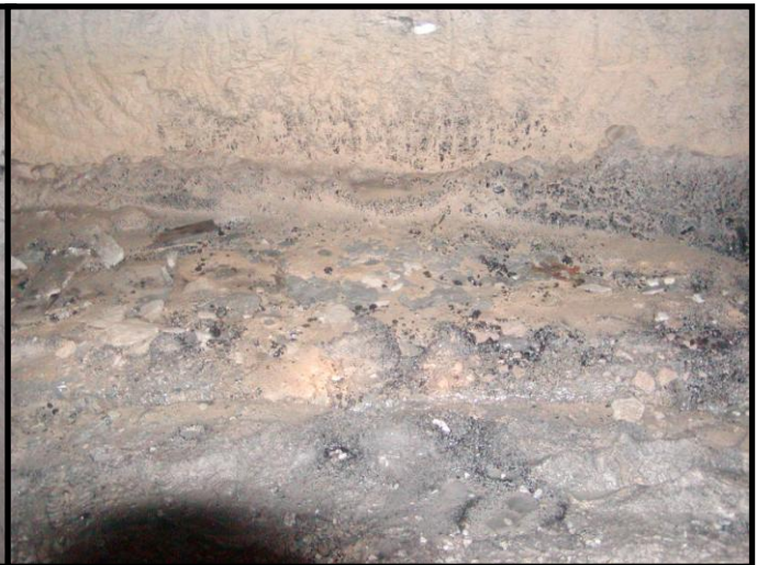
Surface Sediment on Coal Ribs
