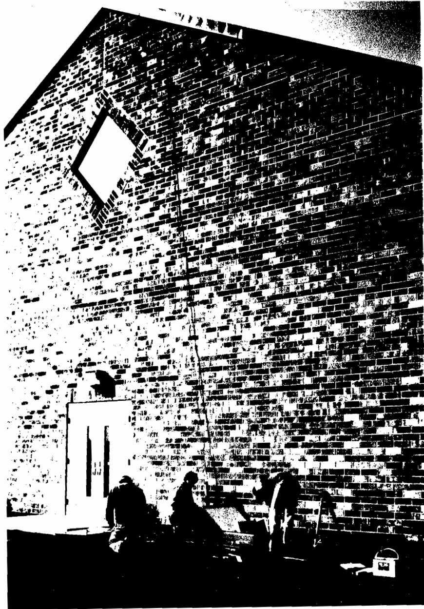
Figure 10.- Structure response transducer and microphone 30-ft high on east wall of St. John's Church
