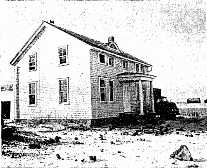
Fig. 1—Building R (after Test R3)
