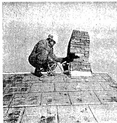
Fig. 10—Chimney damage—building R
