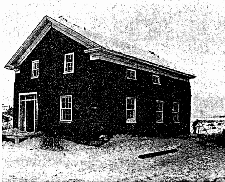
Fig. 2—Building E (after Test E11)
