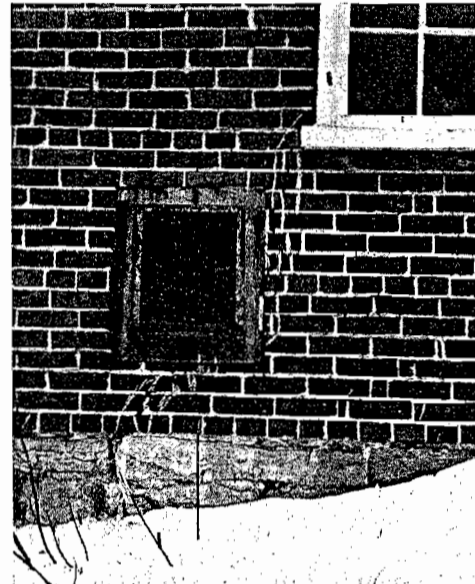
Fig. 6—Vertical crack due to settlement (school)
