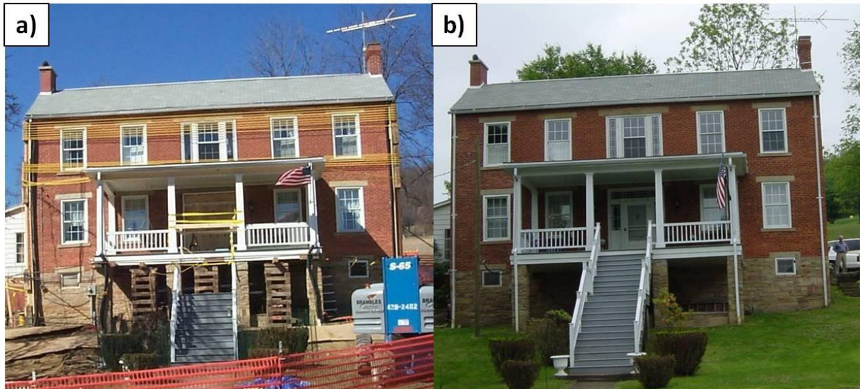
Figure V-18 – Photographs of a) historic farm house in 2001 treated with several mitigation techniques, i.e. banding, cribbing, and trenching and b) farm house on May 21, 2003 (Photograph from PA DEP files).
