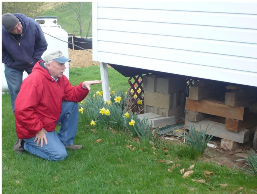
Figure V-17 – Photograph of cribbing (photograph courtesy of N. Iannacchione).
