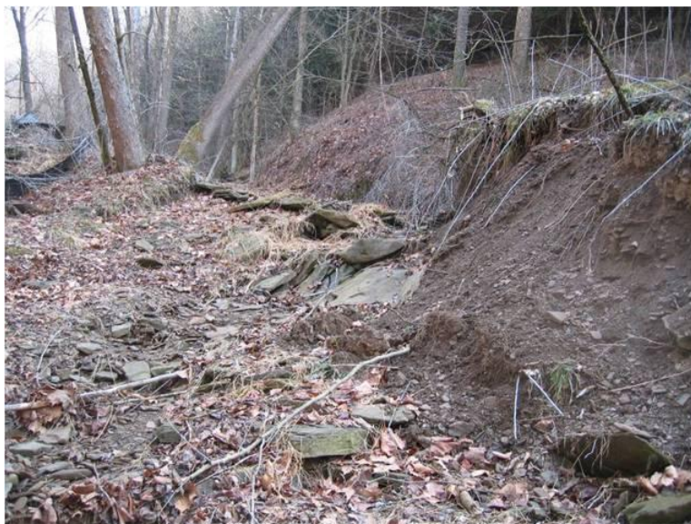
Figure D-4 – Photograph of the post-mining condition of stream 32596. PA DEP agents noted compression ruptures (Photograph from PA DEP files).
