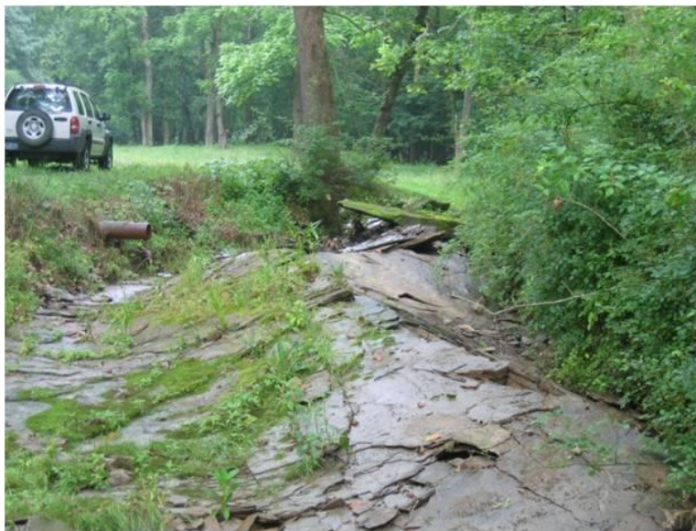
Figure D-3 - Compression rupture observed by PA DEP during a post-mining survey of the 8H panel in Bailey Mine (Photograph from PA DEP files).
