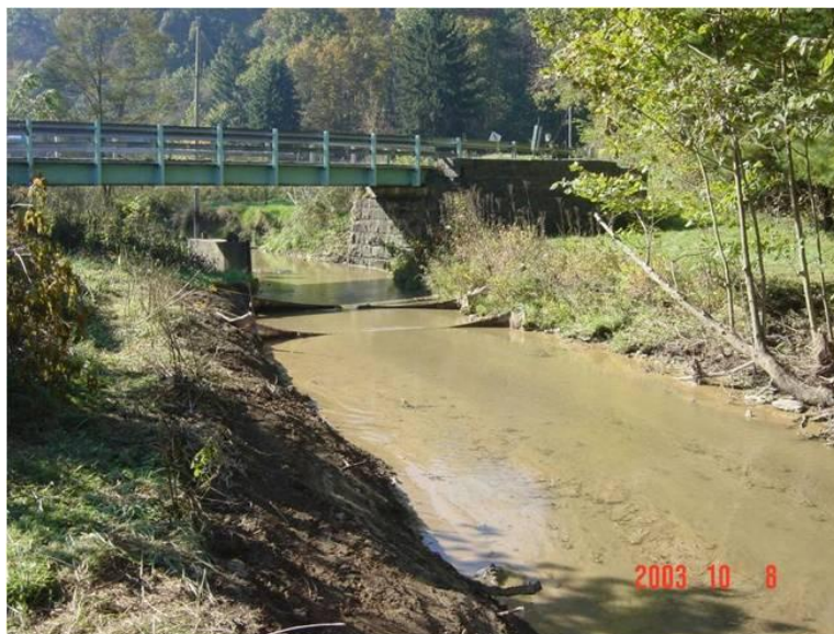
Figure D-8 - Sedimentation observed by PA DEP south of the 8R panel during mitigation work to relieve pooling in the panel (Photograph from PA DEP files).
