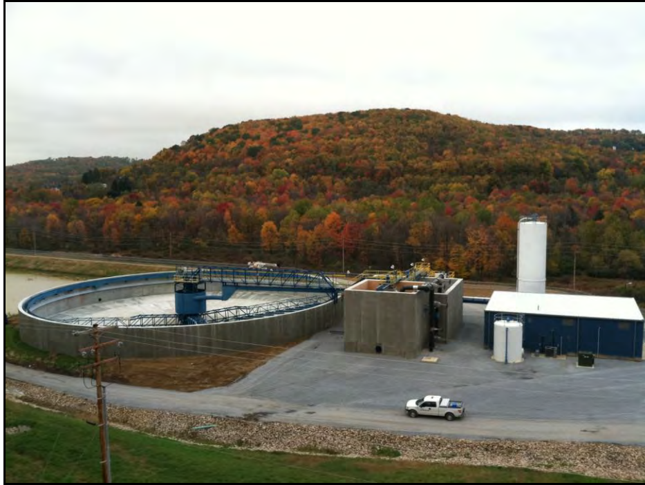
Lancashire 15 AMD Treatment Plant
