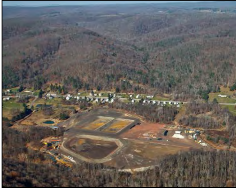
Hollywood Treatment Plant Under Construction –Fall 2010
