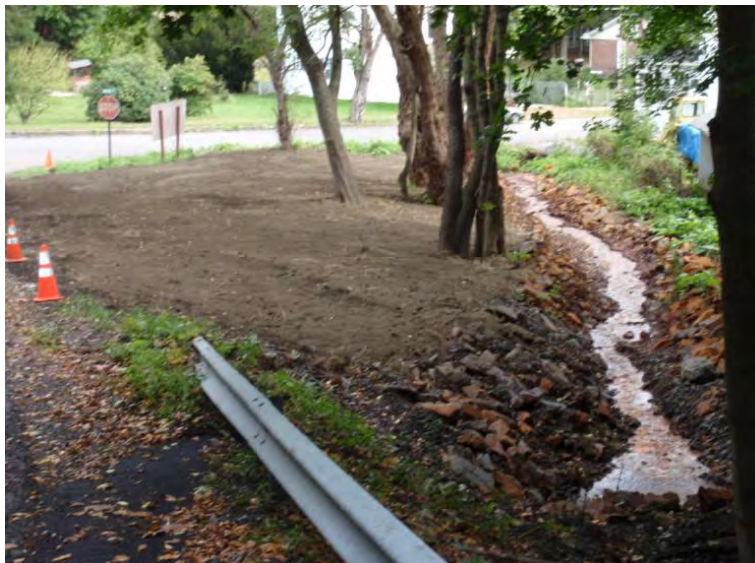
Redefined Clogged Stream To Prevent Further Flooding
