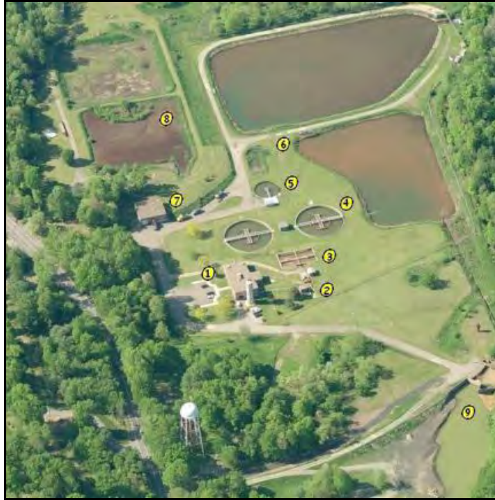
Rausch Creek Mine Water Treatment Plant
