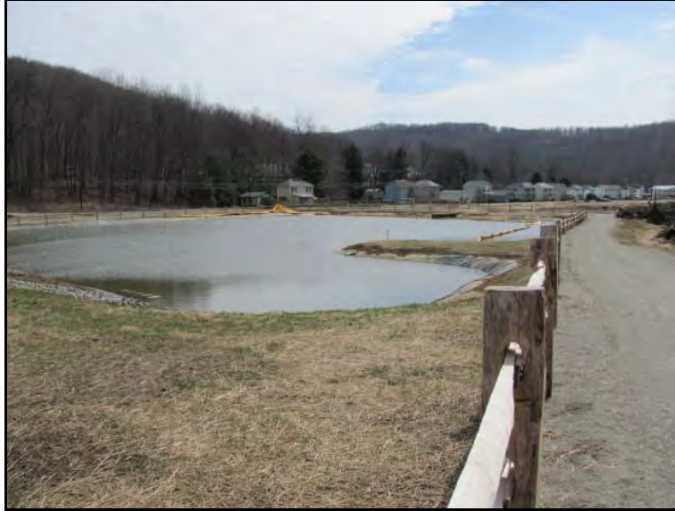
Melcroft AMD treatment facility and public walking path
