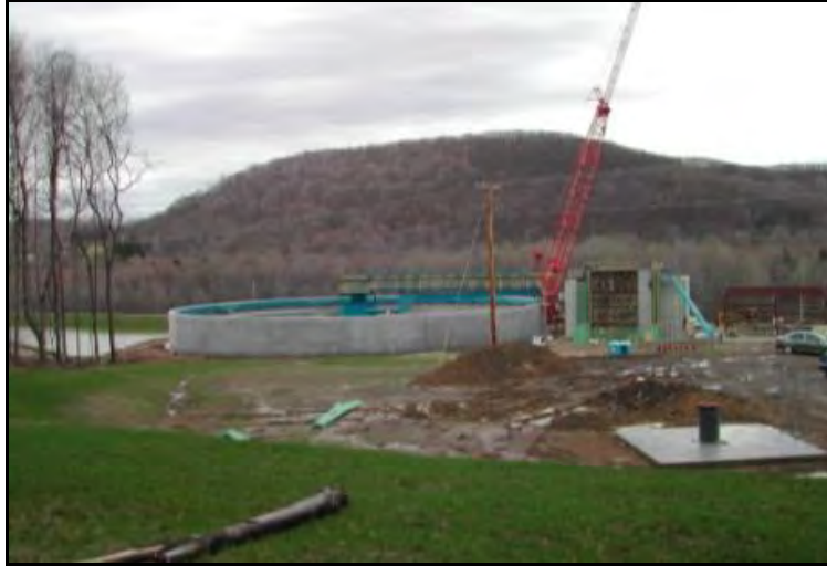
Lancashire #15 Under Construction – Spring 2011
