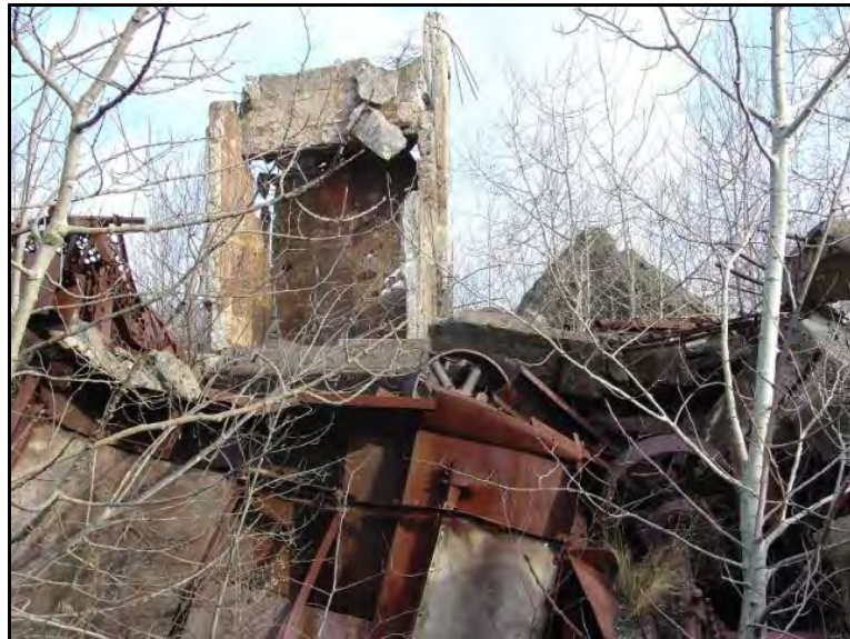
Abandoned Debris at the Taylor Breaker
