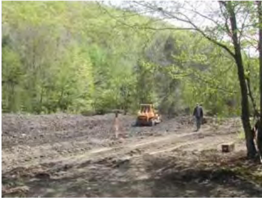
Grading and Surveying – Tyler Impoundment
