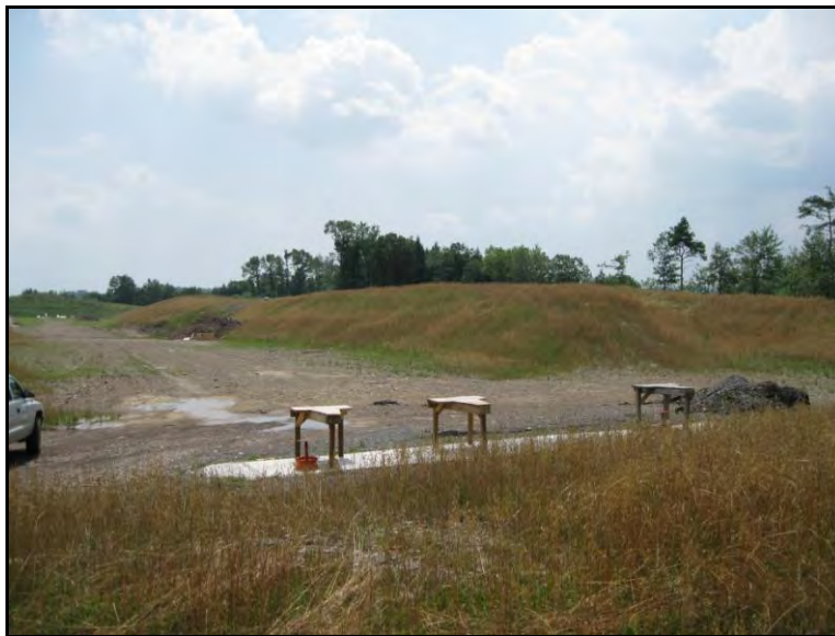
Sportsman's Project – Reconstructed Shooting Range
