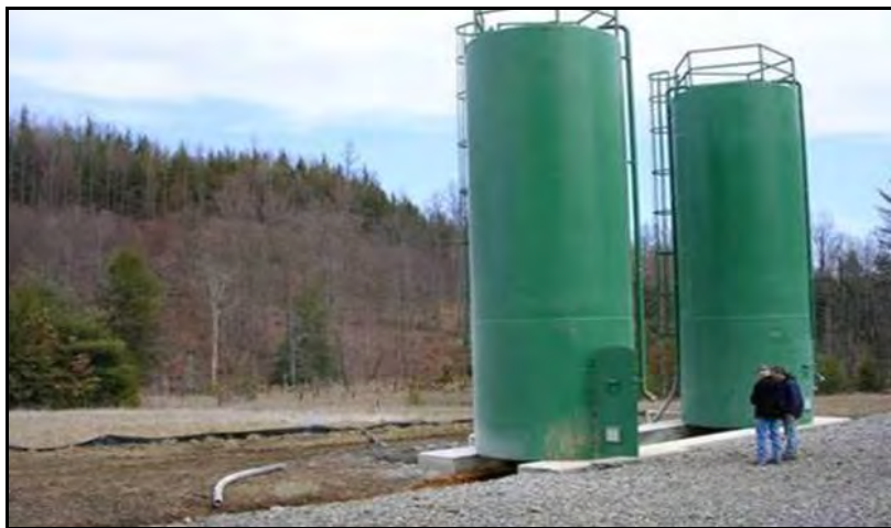
Porcupine Hollow Lime Silos
