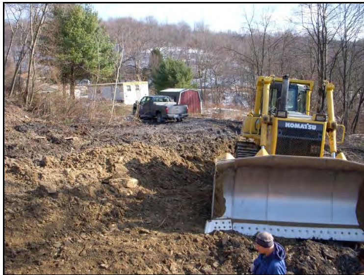
Grading the Pine Creek North Highwall Area
