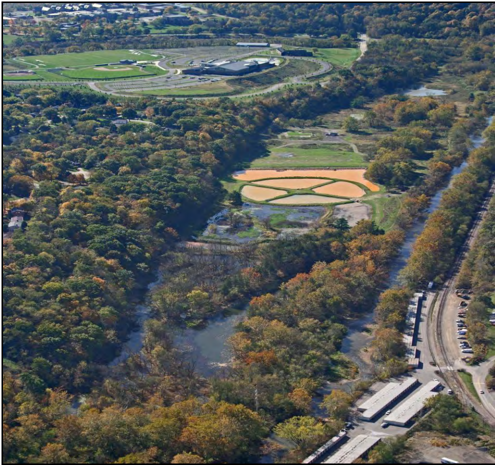
Wingfield Pines Treatment System
