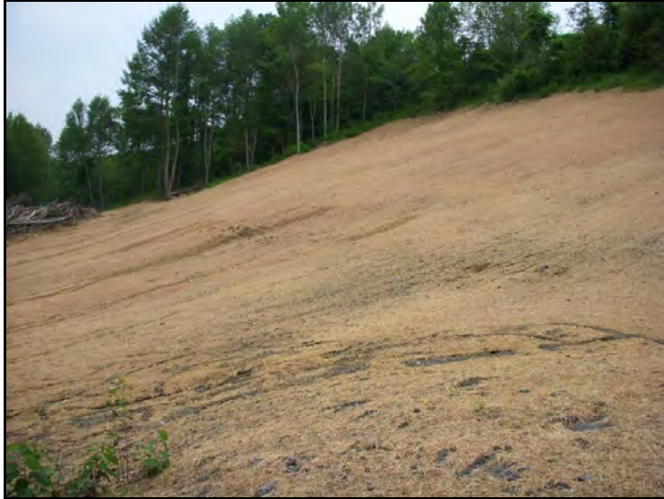
Completed Pine Creek North Highwall Area
