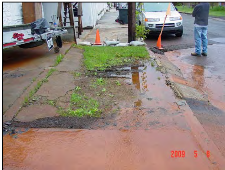
Palo Alto Project Pre-Construction
