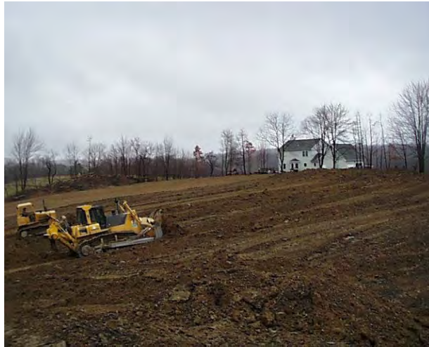
BD Crew backfilling a 3 acre site with 40 foot highwall
