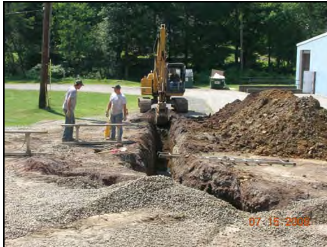
Drain pipe installation Doud's of Plumville
