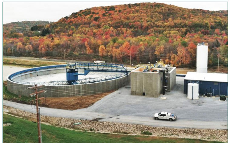
Lancashire No. 15 AMD Treatment Plant
