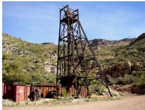
Old headframe at Resolution Mine.
