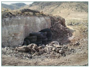
*This is believed to be the first use of toroidal tire plugging in a U.S. mine site.*
