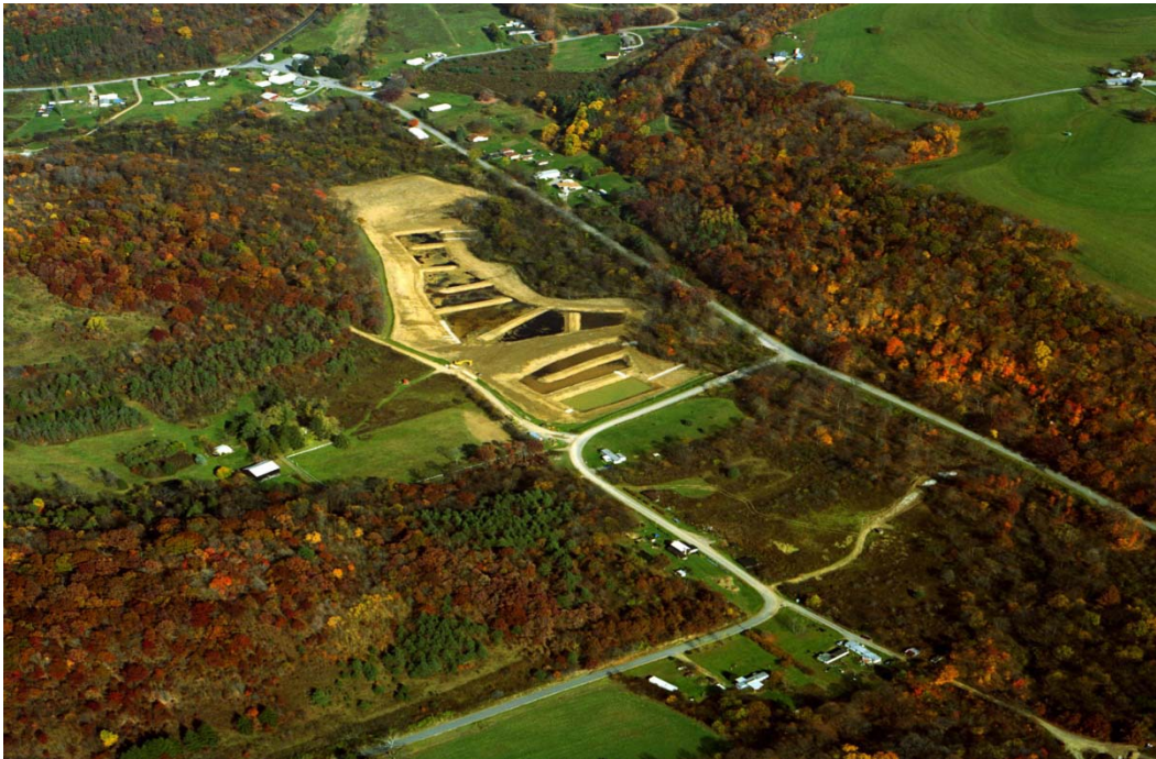
FIGURE 5 – Aerial view of the completed Tanoma Mine Drainage Treatment System.
