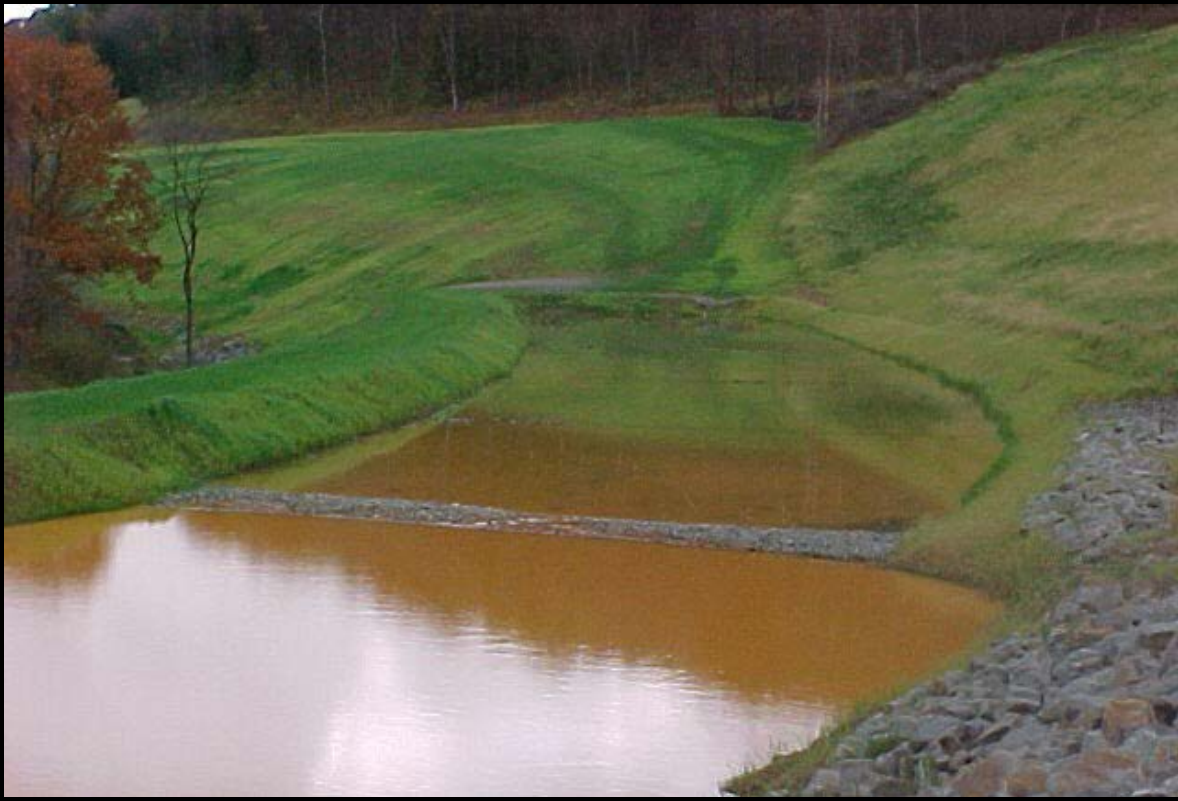
FIGURE 6 – Photograph of the completed passive treatment system and the reclaimed coal refuse pile restored as part of the Sugar Creek Project
