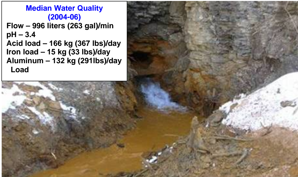
Figure 10. Deep mine discharge in the Caledonia Hollow Tributary impacting the mid-Bennett Branch stream valley, Jay Township, Elk County.
