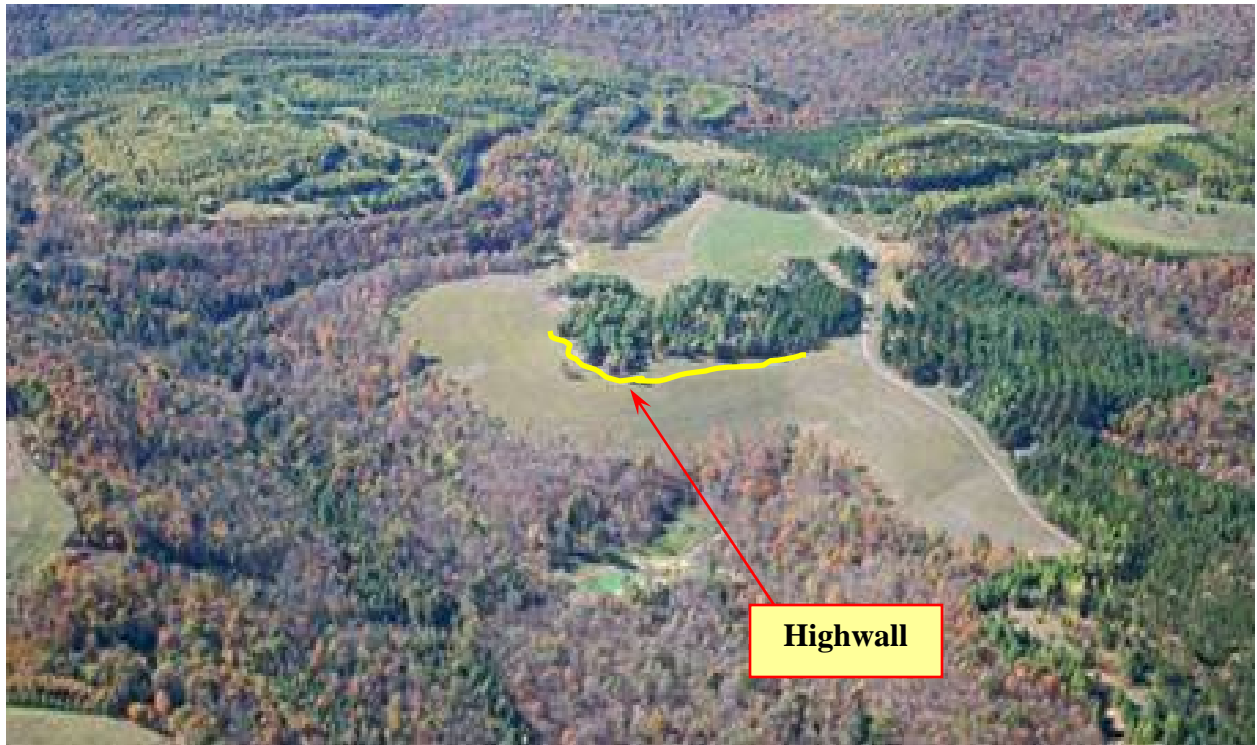
Figure 18. Aerial view of the same abandoned surface mine on State Game Lands No. 311 in Benezette Township, Elk County, following reclamation.
