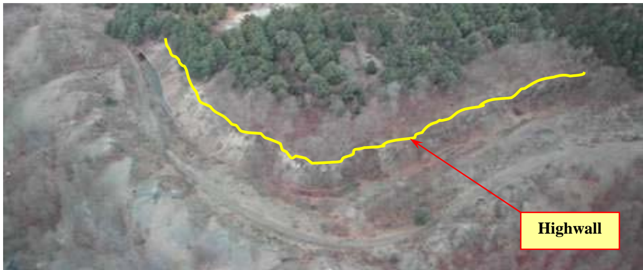
Figure 17. Aerial view of an abandoned surface mine on State Game Lands No. 311 in Benezette Township, Elk County prior to reclamation.
