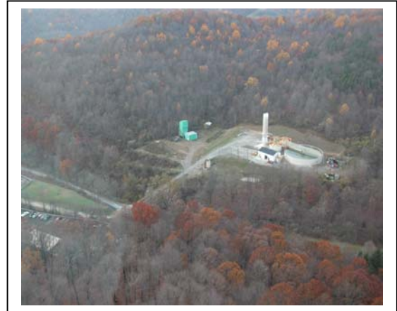
Shannopin Treatment Plant
