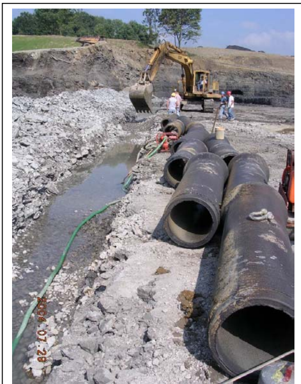
July 2004 Drain Construction
