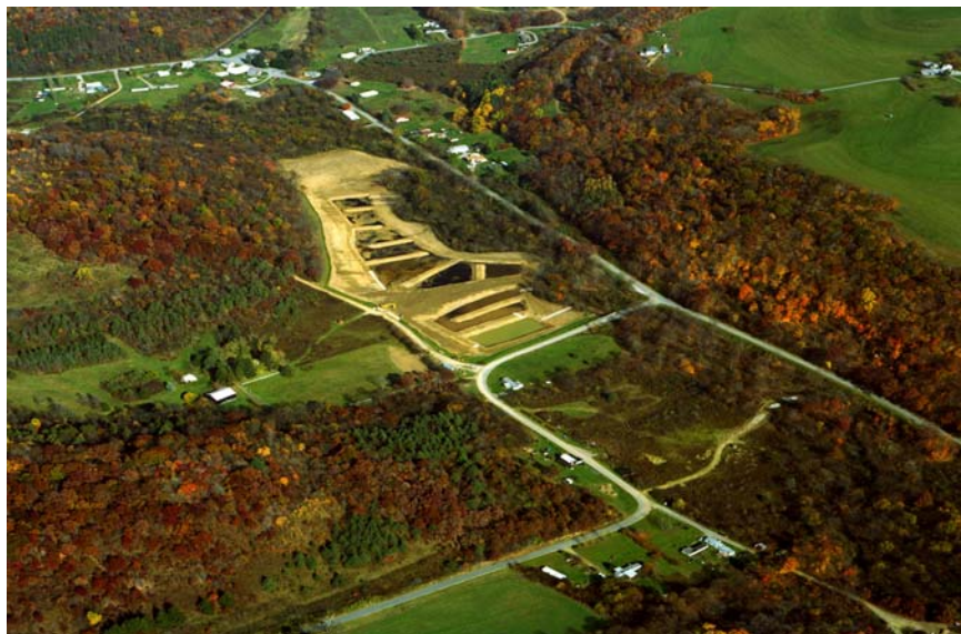
Aerial view of the completed Tanoma Mine Drainage Treatment System
