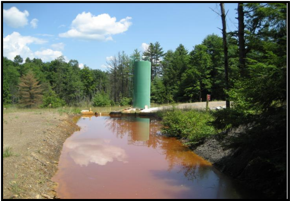
Figure 15 – Elk cooling off in COE passive treatment system PA 3888 (above), tipping bucket lime doser treating AMD Discharge No. 17 PA 1934 (below) photos from PGC website
