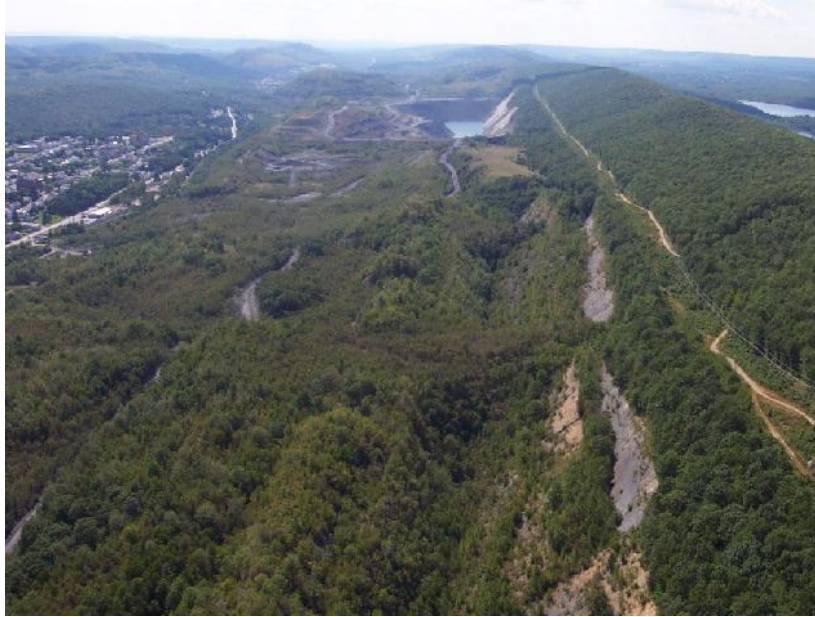
“Highwall” Exposures in Panther Valley - PA DEP BAMR
