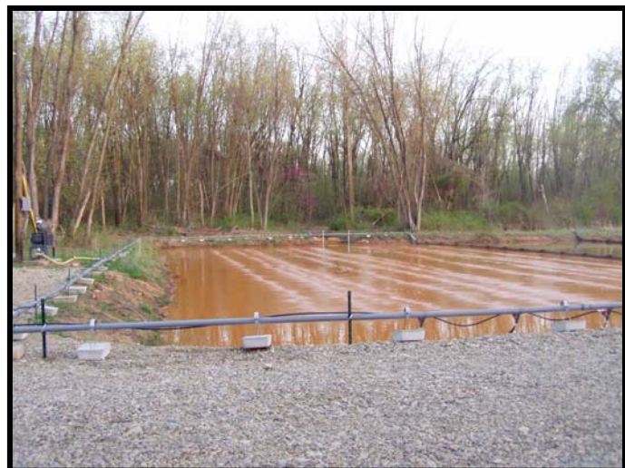
Figure Lasaire-12. Lasaire Aeration System at the Upper Latrobe Borehole.
