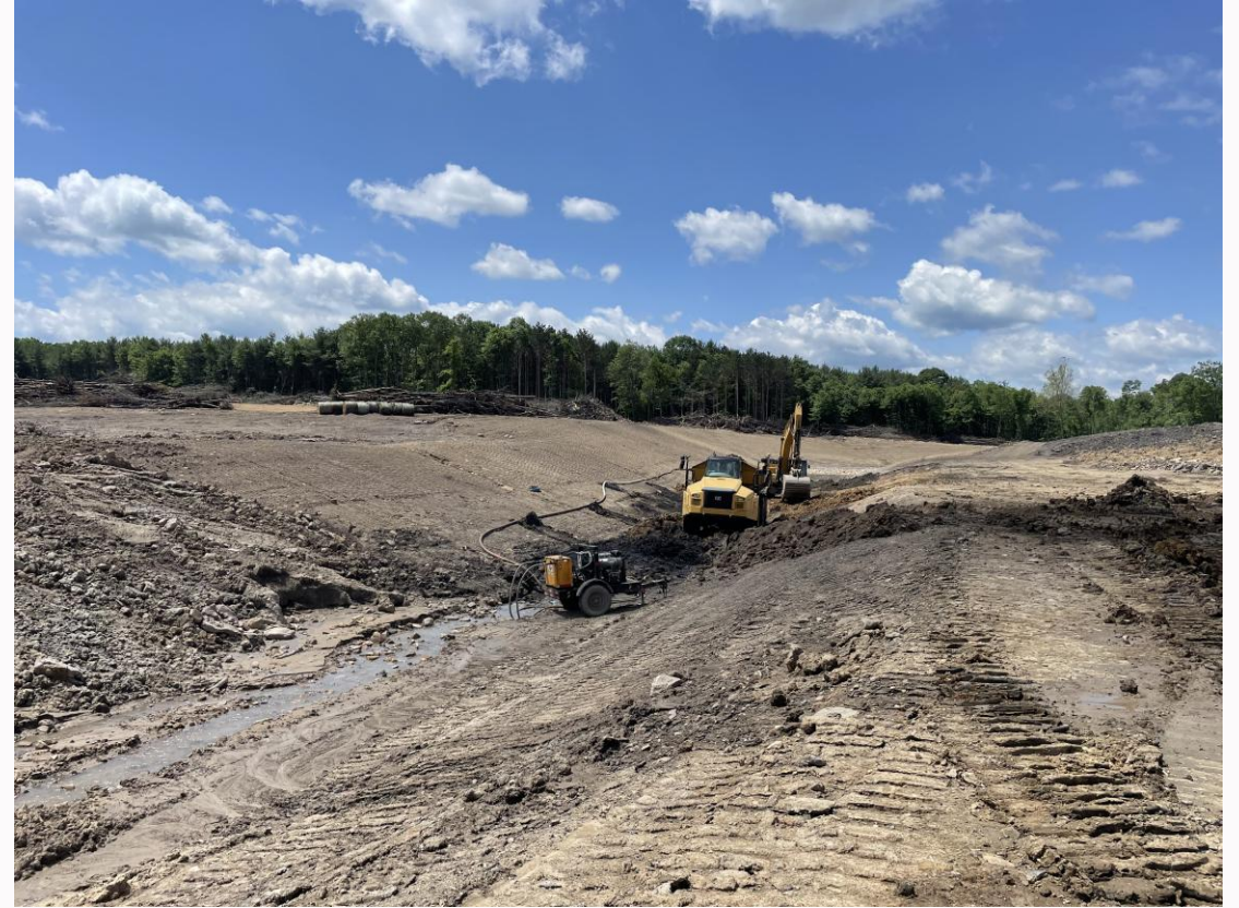
Stream Channel Excavation with Bypass Pumping
