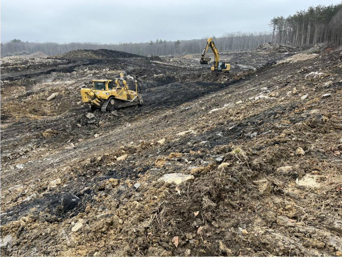
Stream Channel Excavation
