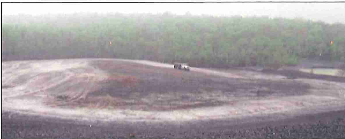
Applying Ag-Lime on Reclaimed Refuse Bank May 2014 – PADEP BAMR
