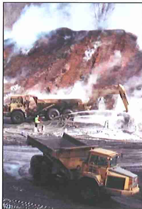
Spraying Foam on Hot Refuse, March 2014 – Scranton Times-Tribune
