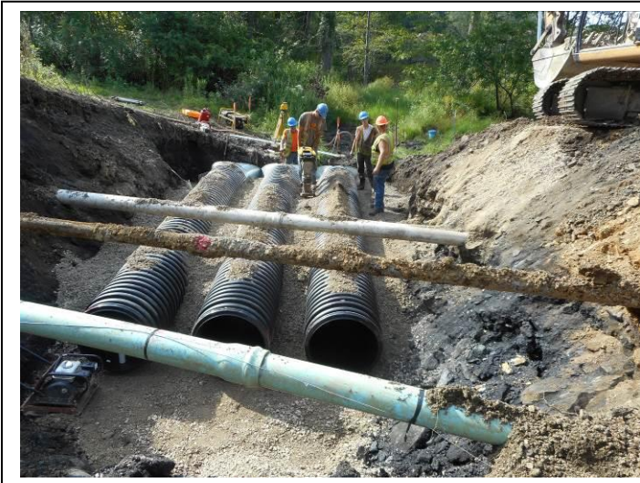
Installing the three 36-inch pipes under the utilities.
