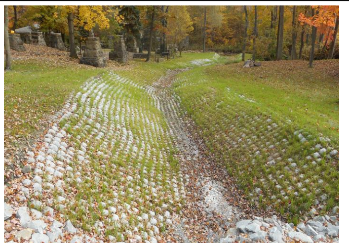
Block erosion block channel.
