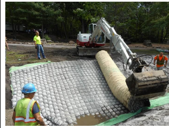
Installing block erosion control matting through the park.
