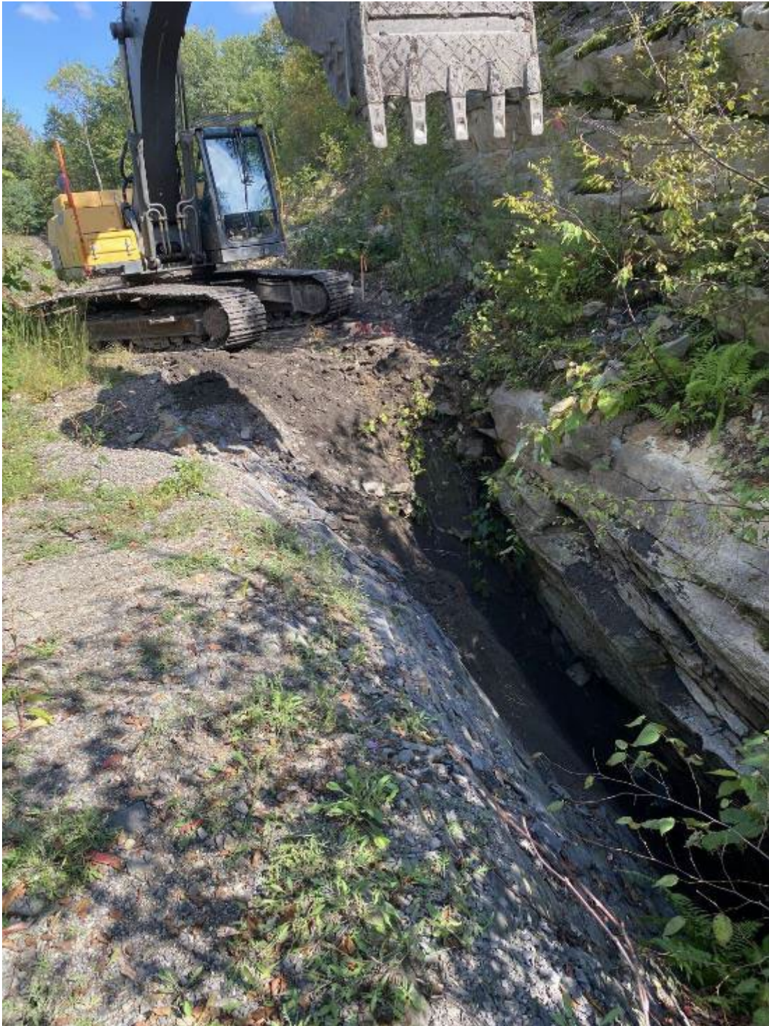
Backfilling the No. 1 Slope
