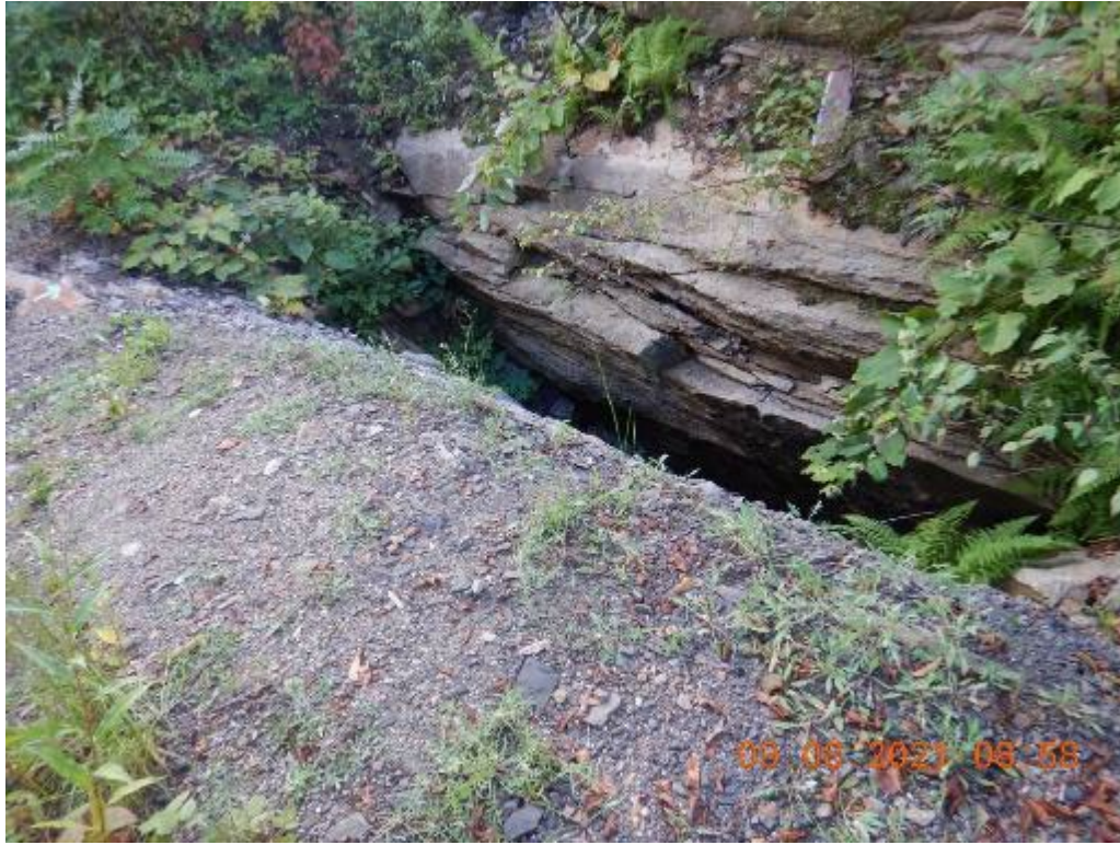
AML Feature 2065-05, the No. 1 Slope opening, looking Southeast
