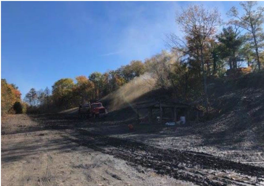
Mulching of Grading Area and No. 1 Slope
