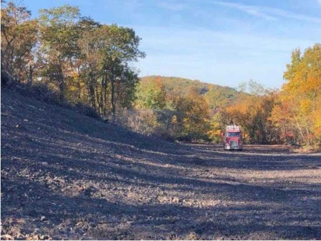
Mulching of Grading Area
