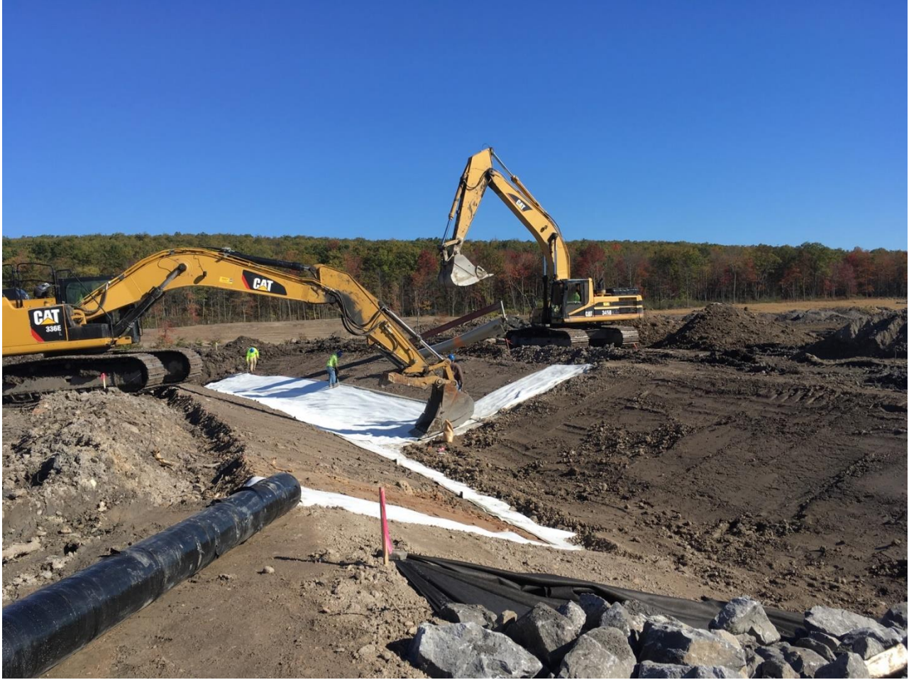
Installing Ditch G
