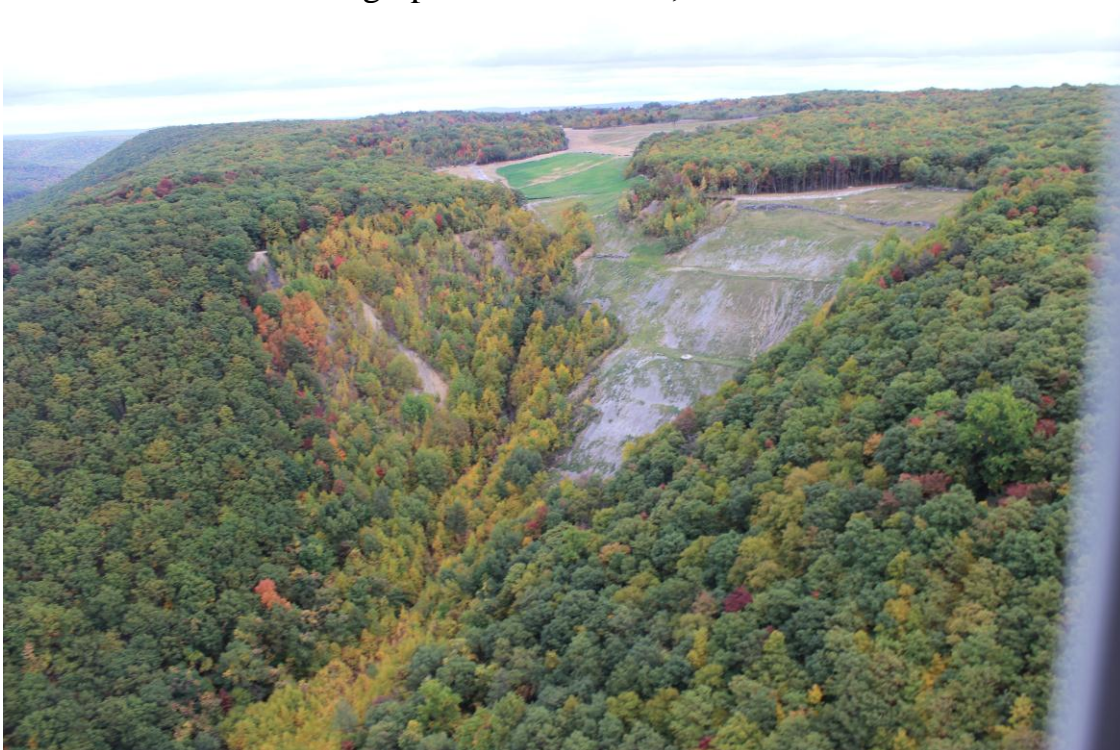
Aerial Photograph of the “Wash”, Post Construction
