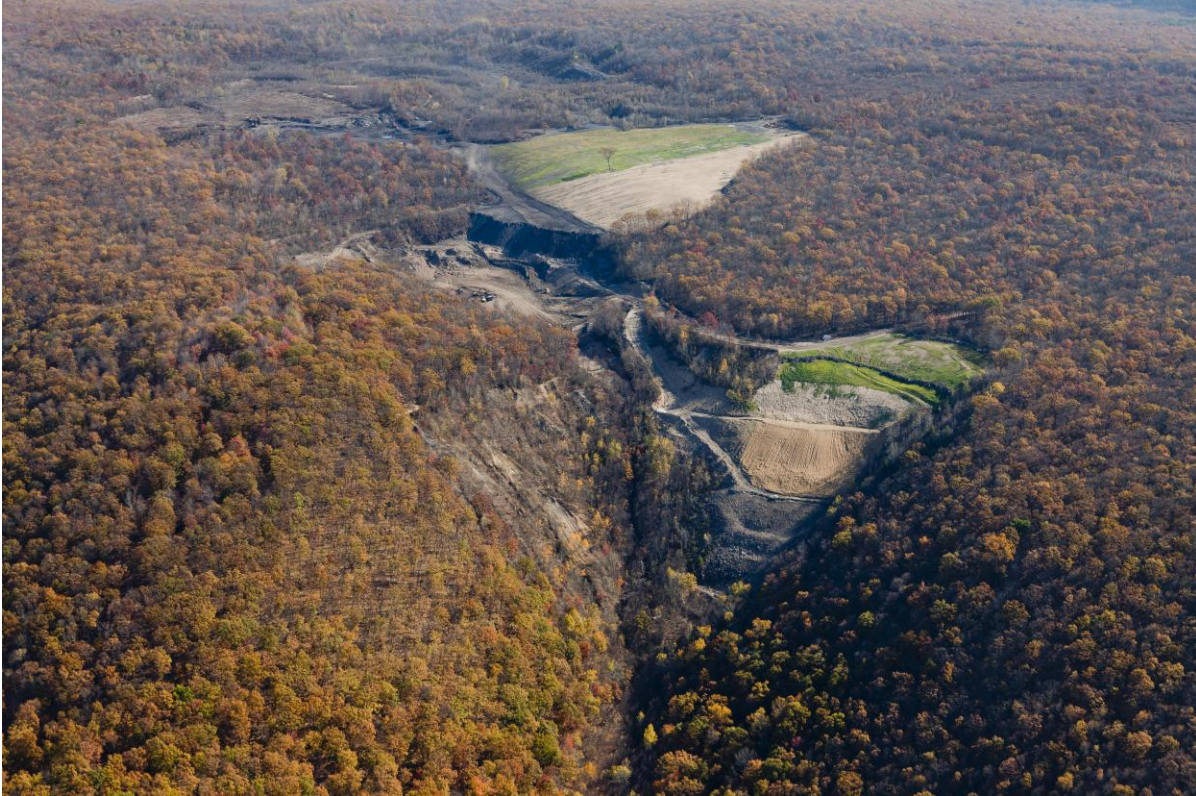
Aerial Photograph of the “Wash”, During Construction
