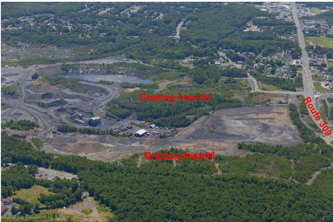
Looking south at Borrow areas, Grading Area #3 and #4
