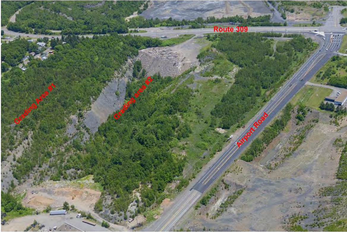
Photo of Dangerous Highwall #1 looking to east.
