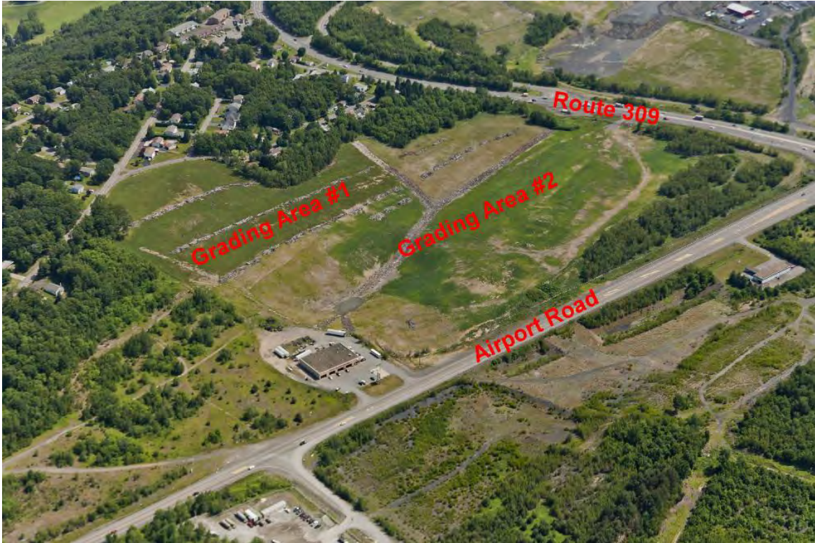
Reclaimed Dangerous Highwall #1 looking to the east.
