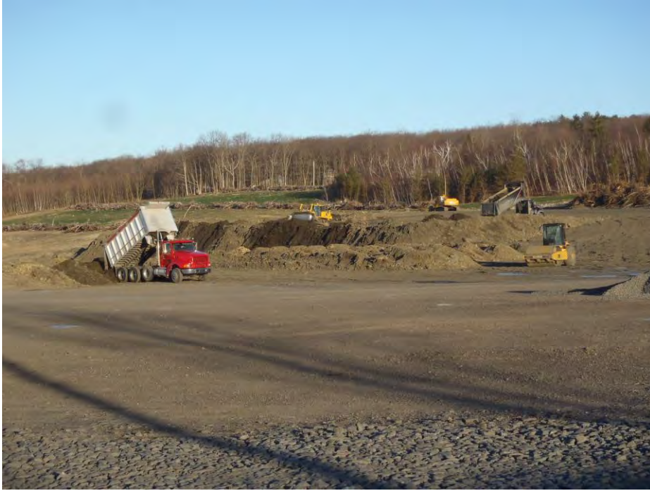
Backfilling of Dangerous Highwall #1 looking northwest.
