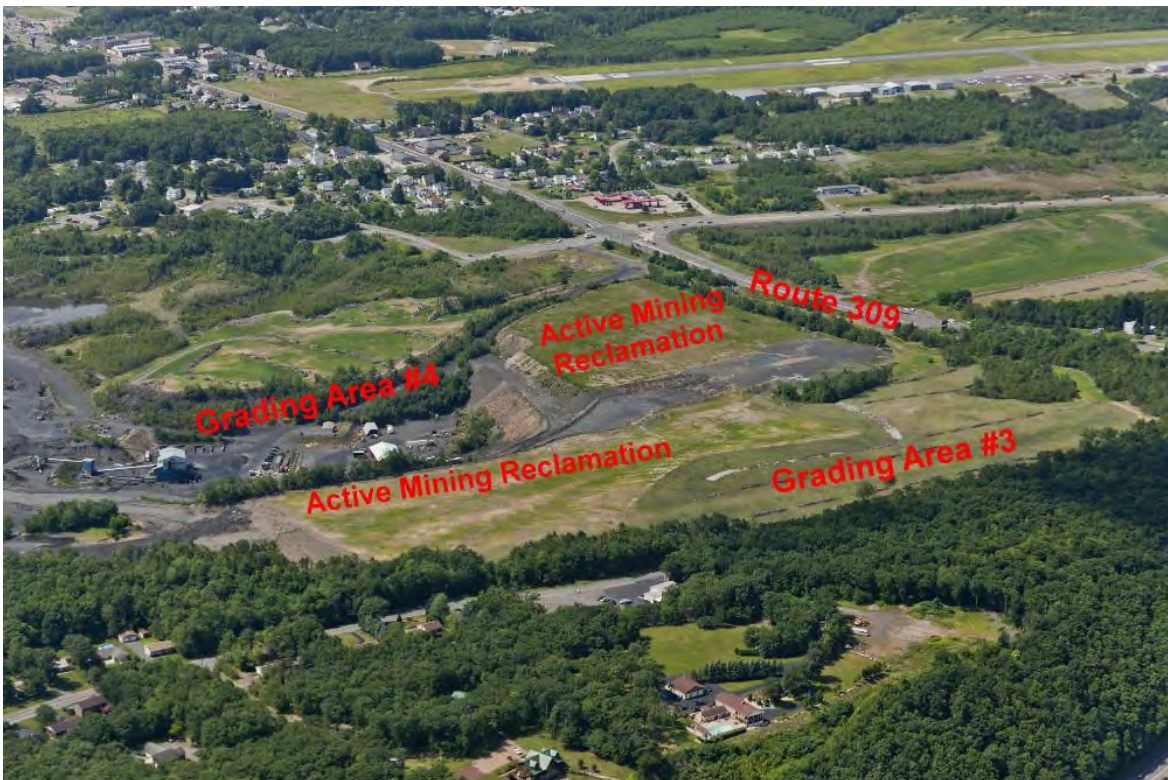
Looking south at Reclaimed Borrow areas, Grading Area #3 and #4
