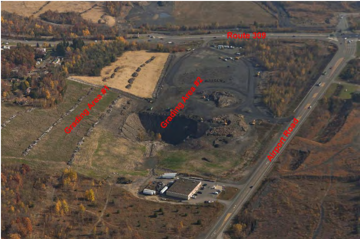
Photo of Dangerous Highwall #1 looking to the east.
