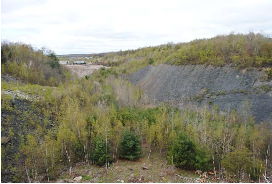
Photo of Dangerous Highwall #1 looking to the west.
