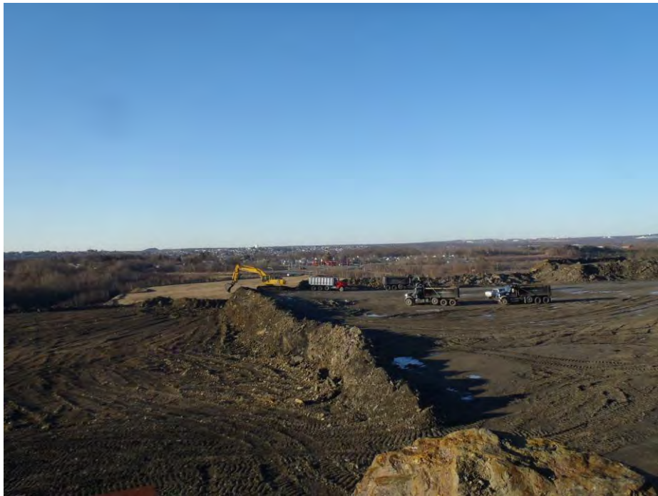
View south at excavation of Grading Area No.3.
