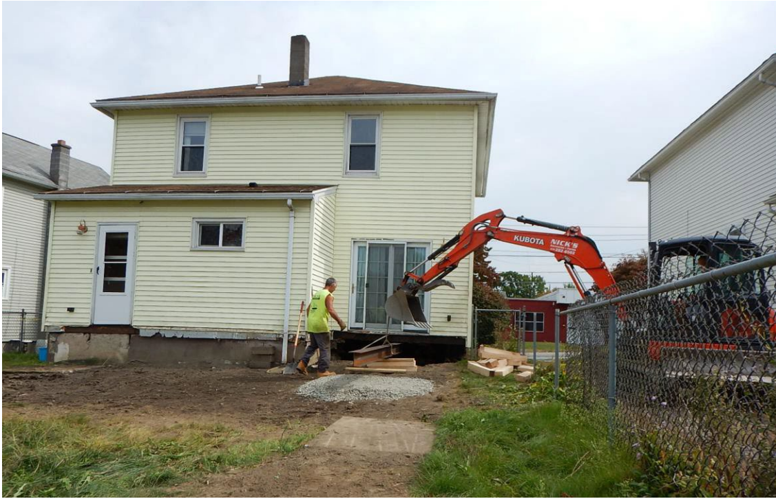
Installation of a 40-foot-long steel I-beam under the home.
