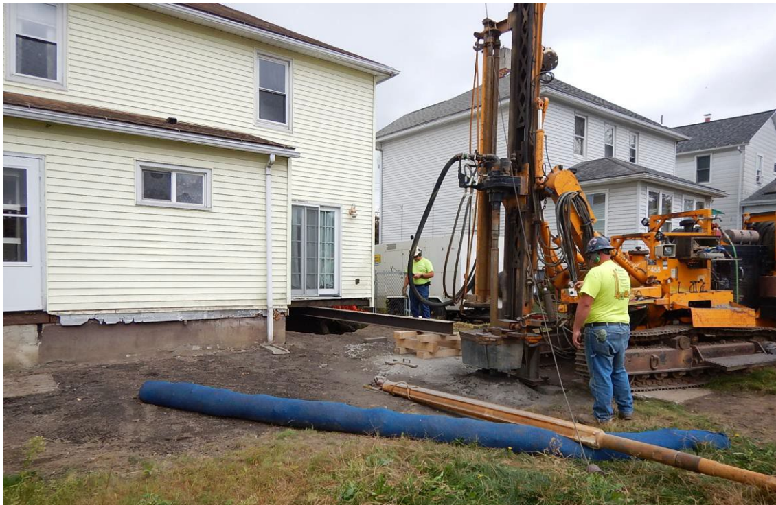
Drilling exploratory borehole in backyard
