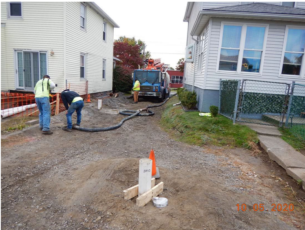
Fill material injection of borehole
