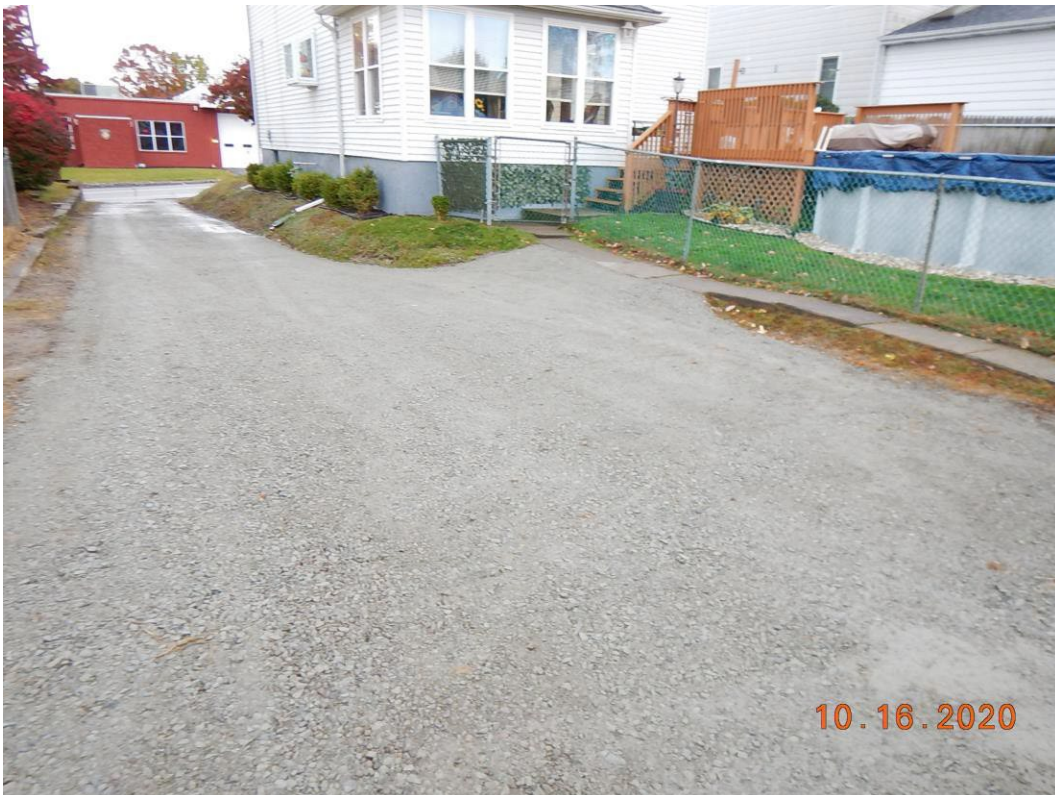
Driveway restored with 2A modified stone
