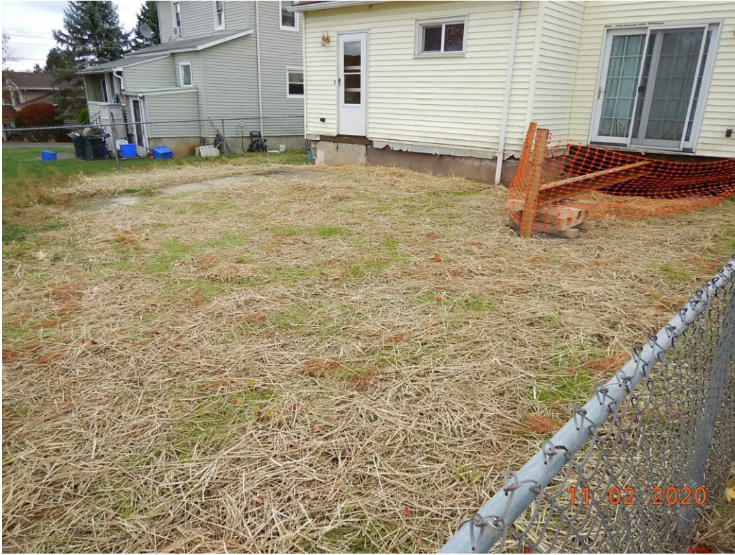
Backyard restored; steel beam remains in place
